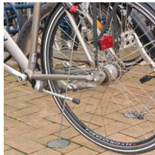
In Odense butterfly racks have been supplemented by a locking mechanism in the shape of a wire pulled up from the ground.
