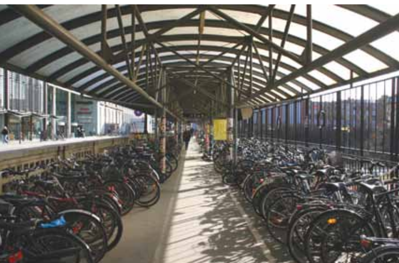
Capacity was doubled at the Aarhus railway station by replacing 500 ordinary perpendicular, front wheel spaces with 1000 two-tier spaces.
