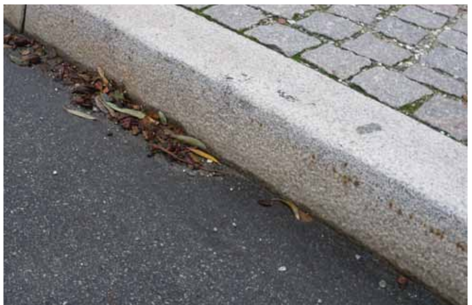
The traditional Danish cycle track with a kerb provides excellent segregation between road user groups.
