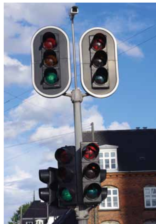
Right turn lane with separate phase for turning motor traffic used to stop bicycle traffic going straight ahead, but with radar detection cyclists are now only stopped when there actually are vehicles in the right turn lane. Amager Boulevard, Copenhagen.
