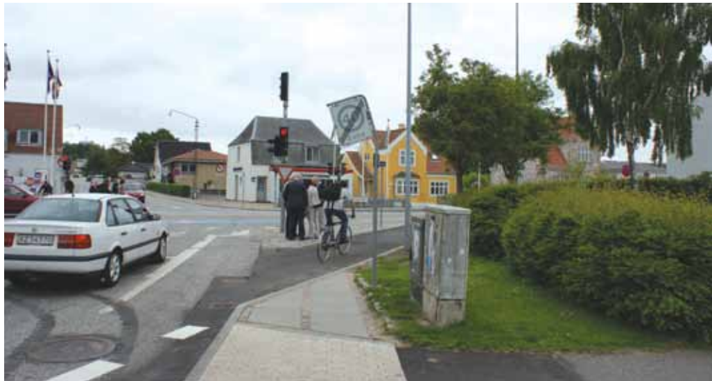
Shunt in Aalborg improves passability since cyclists needn't wait for the green signal before turning right.
