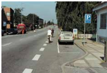
The parking bays here are too narrow. A car door is 0.9 m wide.
