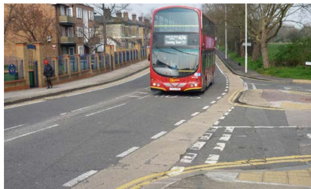
Dashed markings and coloured surfacing used for cycle lane
