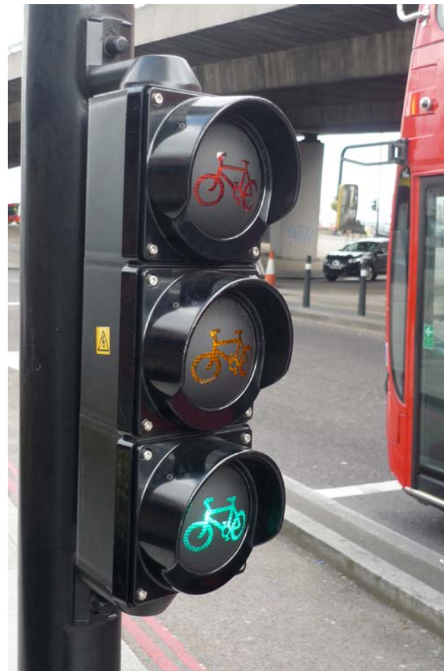
Detail of low-level cycle signal
