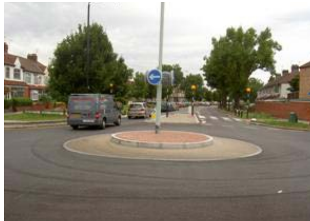
Compact roundabout in UK with overrun strip
