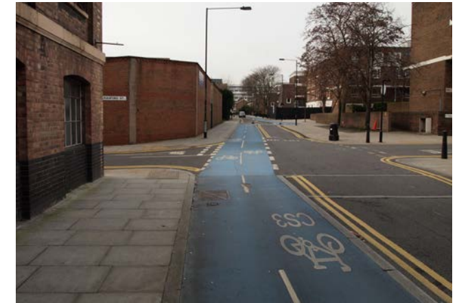
Two-way track continued across priority junction without deviation in a traffic calmed street – Cable Street, Tower Hamlets
