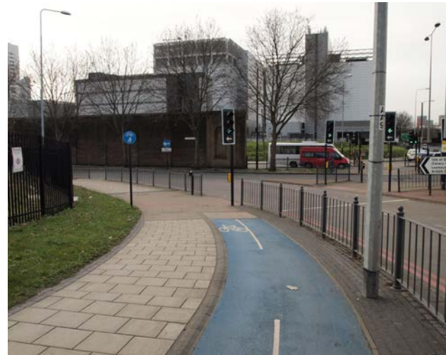
Toucan crossings are often used to carry off-carriageway tracks through or around junctions
