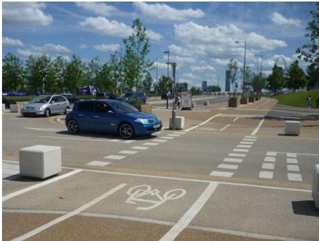
Bent-out cycle tracks with priority at Waterden Road, Hackney. Note that elephants' footprints should not be used to mark this kind of crossing
