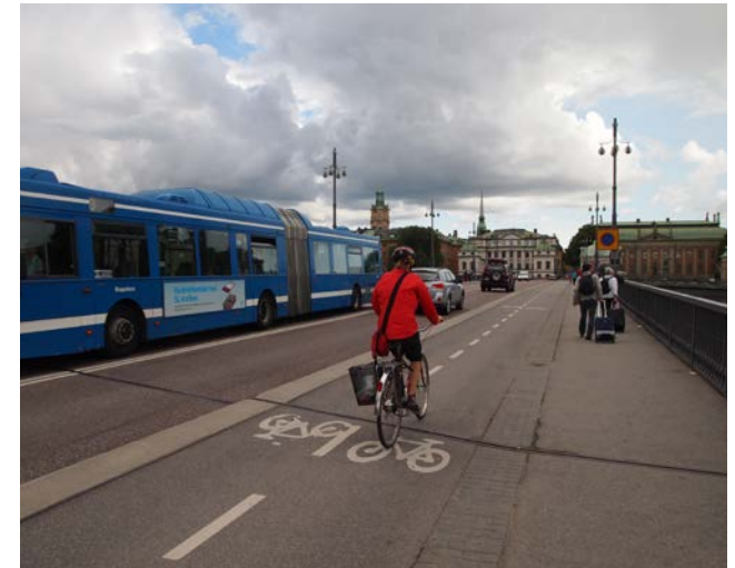
Segregated lanes/tracks with low kerb upstands – in Utrecht (left) and Stockholm (right)
