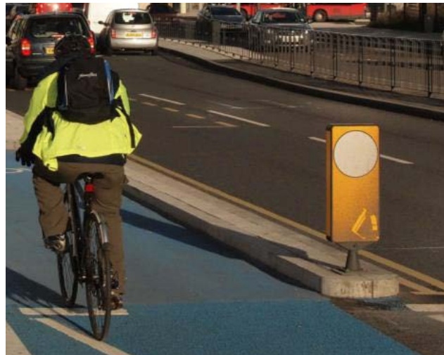
Blank bollard (without recommended clearance)
