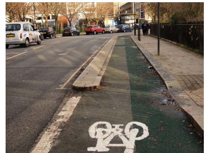
Skinner Street, Islington: battered kerbs and gaps to allow for uncontrolled pedestrian crossing
