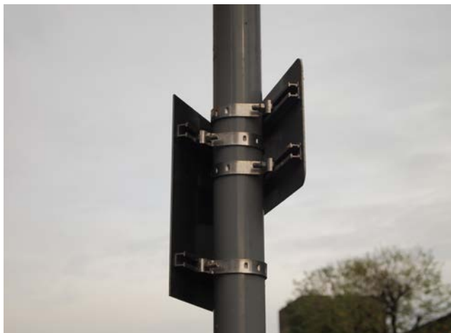
Signs with fixing channels and mounting clips
