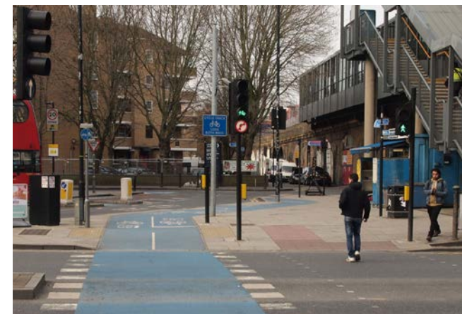
Red blister tactile paving used at controlled crossings. Note the buff blister tactile at the uncontrolled crossing of the cycle tracks, bottom
