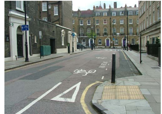
Footway build-out with contraflow cycle provision
