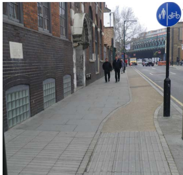
Ladder and tramline at 2400mm depth (left) and 1200mm (right)
