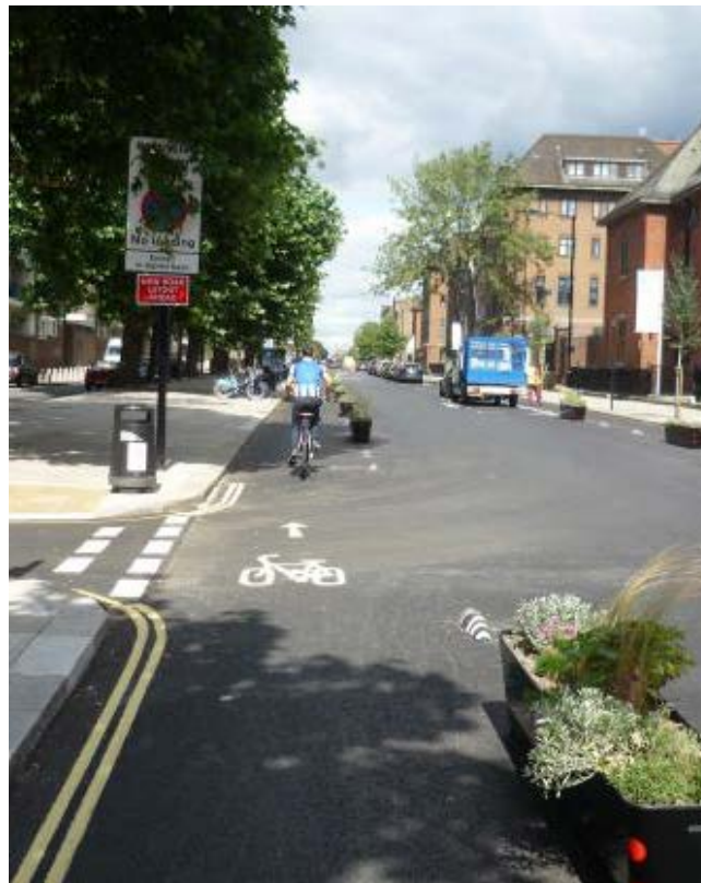
Flexibility of infrastructure at Royal College Street, Camden has allowed for adjustment of lane widths and relatively easy replacement of damaged separators and planters
