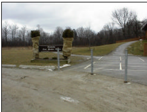
Example of Bollards – City of Brampton
