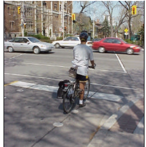
Bicycle Detector Dots – Toronto, Ontario
