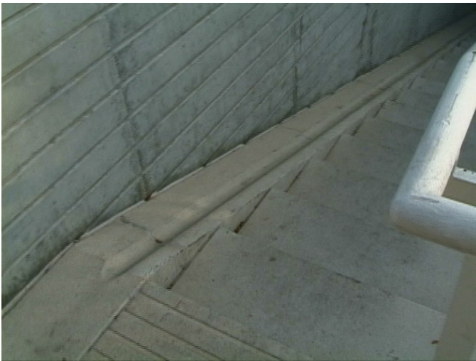
Channel for bicycle wheel in concrete staircase at McDonald's Cycle Centre, Chicago.
