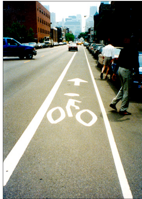
Figure 7-12: Proper use of a bike lane symbol
