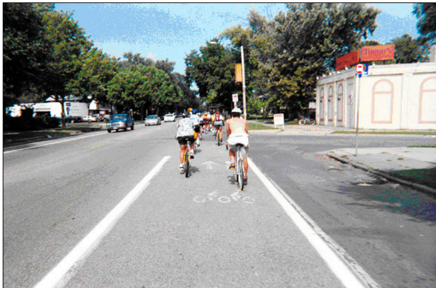
Figure 4-11: Bicycle Lane on a Roadway with Curb but No Gutter
