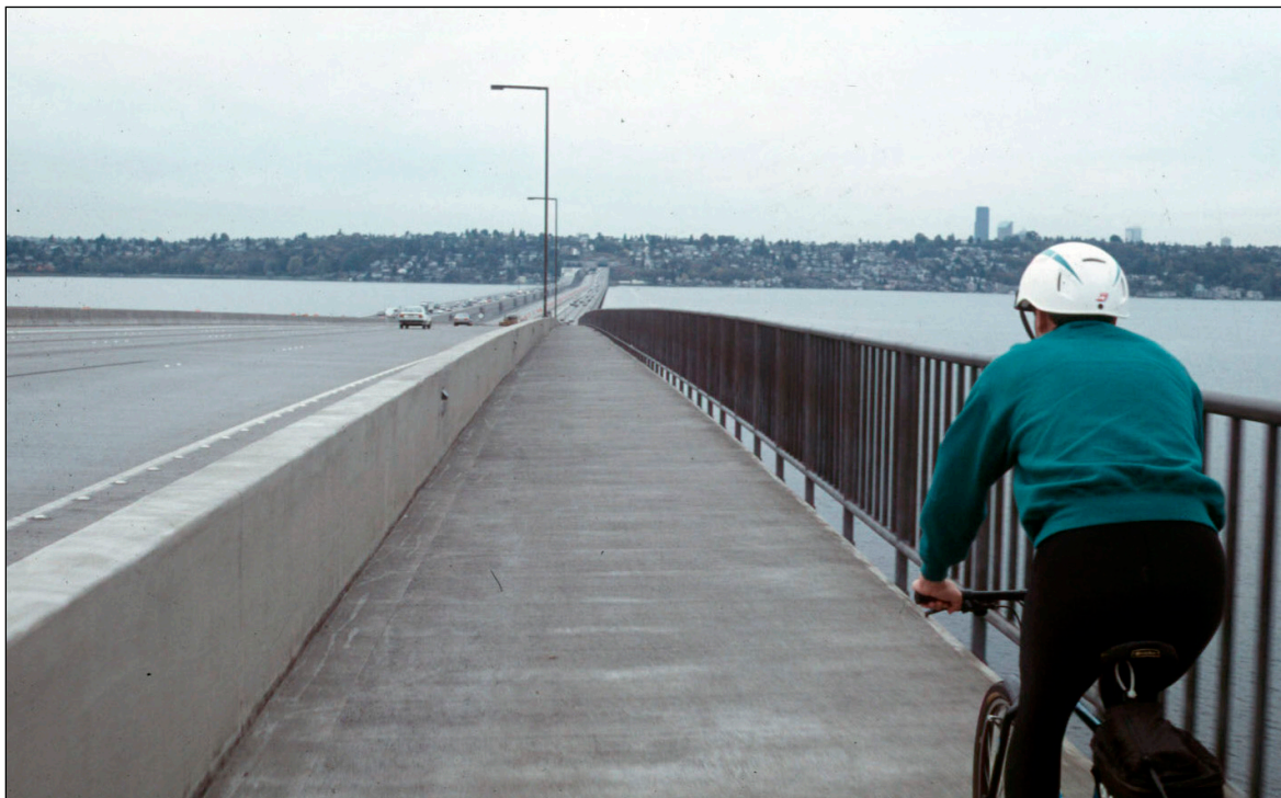
Figure 4-6: Bikeway with a Jersey Barrier-Protected Shoulder, Seattle Picture courtesy of www.pedbikeimages.org / Dan Burden
