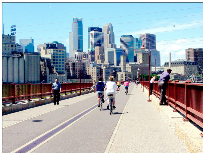
Figure 1-1: The Stone Arch Bridge into downtown Minneapolis was one of Minnesota's first Transportation Enhancements projects, and is a key link in the city's planned bicycle freeway system
