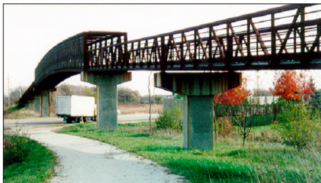
Figure 6-3: Example of creative use of an overpass for non-motorized users
