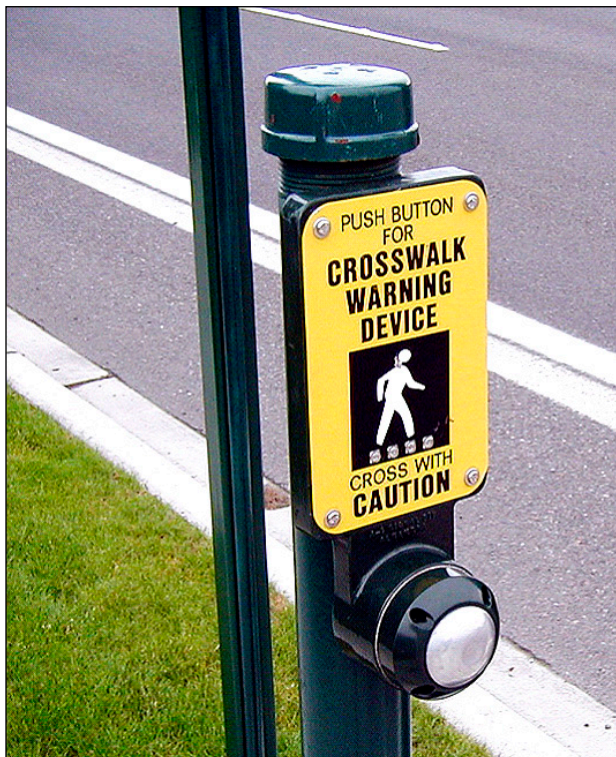
Figure 7-11: Example of an accessible crosswalk push button
