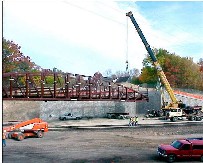
Figure 2-3: Mn/DOT and the Department of Natural Resources coordinated on a road construction project that involved constructing a bridge for the Luce Line State Trail
