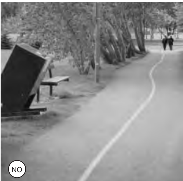
Figure 1-4: This shared-use path includes a number of hazards intruding into the necessary “comfortable lateral clearance.”
