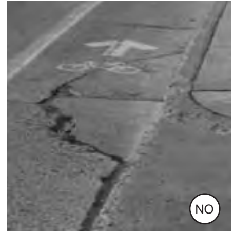
Fig. 3-11: Serious pavement cracks in a bicycle lane can cause a bicyclist's front wheel to turn, resulting in a crash.
