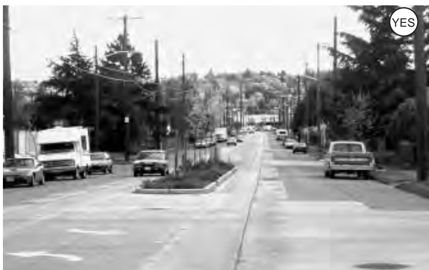
Figure 2-31: Designers replaced 4 through lanes on this narrow road with 2 through lanes, a center turn lane, and space for bicyclists.
