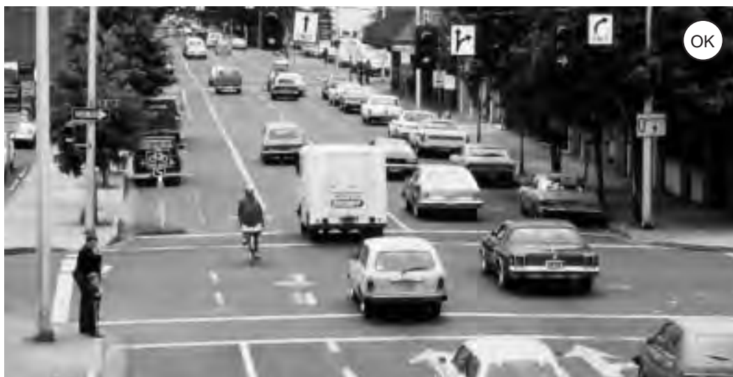
Fig. 3-6: In special situations, bicycle lanes on the left (like the one shown) can work. But in most situations, bicycle lanes on one-way streets should be on the right, rather than the left.
