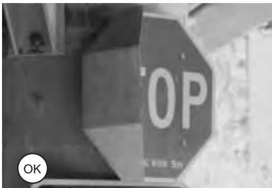
Figure 4-77: Where there is no alternative, a shield may be used to keep motorists from seeing a sign for path users.
