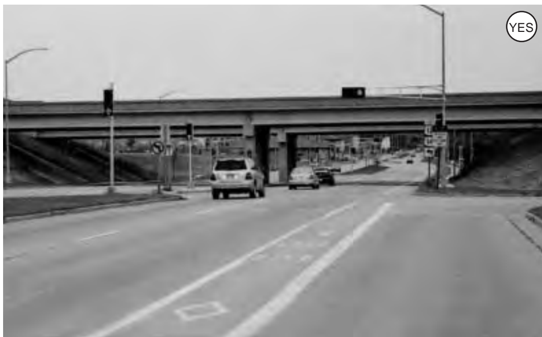
Figure 3-44: An urban-style interchange design is easier for bicyclists to negotiate than a rural-style design with its high-speed merges and broad sweeping curves.
