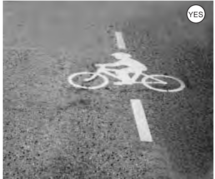
Figure 2-52: Close-up of Madison-style loop detector pavement marking.
