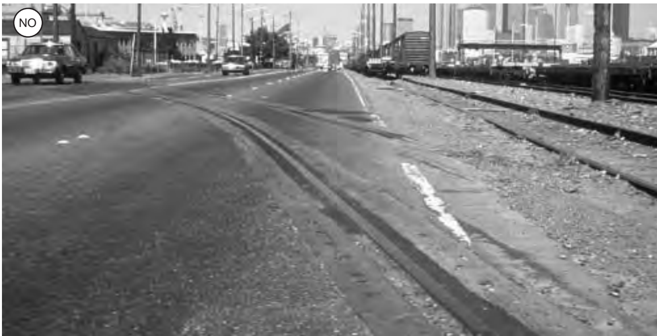
Fig. 2-38: An old unused diagonal railroad crossing. The flangeway can catch and turn a bicyclist's front wheel, especially when wet, and the roughness can also cause a tumble.
