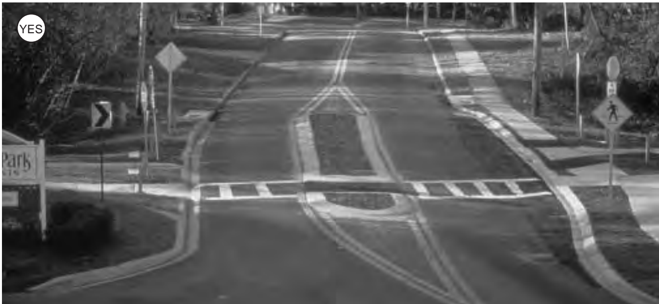
Figure 4-99: Traffic calming measures can make a significant difference in how easily path users can get across a roadway.
