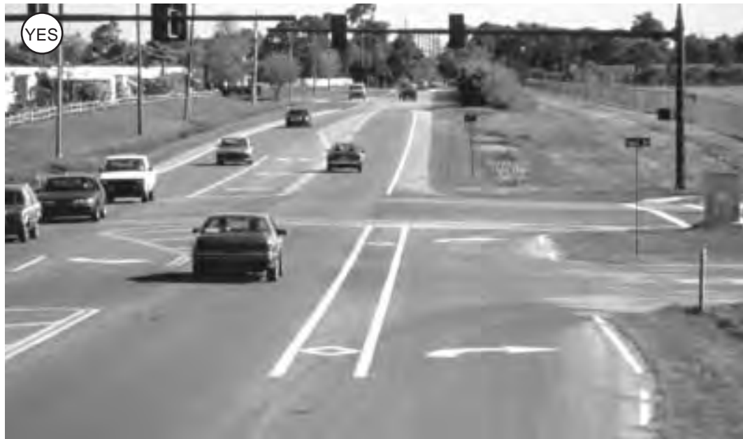
Figure 3-37: This intersection features a bicycle lane to the left of a right-turn lane. Note how it lines up with the bicycle lane on the far side of the intersection.
