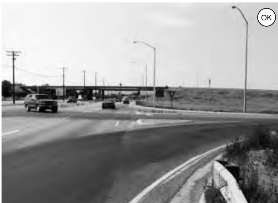
Figure 3-45: Interchanges with high-speed turns and merges are suited only to an environment that will remain rural.
