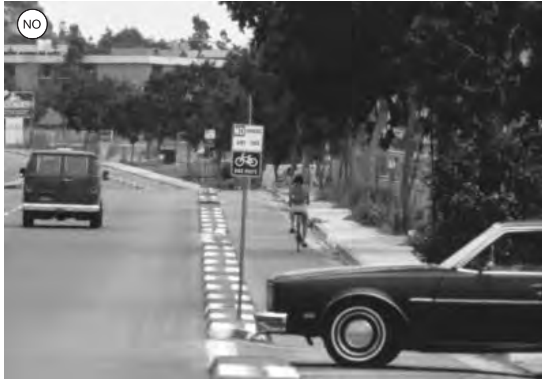
Figure 3-10: With few exceptions (e.g., contraflow bicycle lanes), barrier-delineated bicycle lanes create more problems than they are intended to solve. For example, they hamper bicycle and motor vehicle turns and motorists exiting from a cross street or driveway can easily block a bicyclist's passage.
