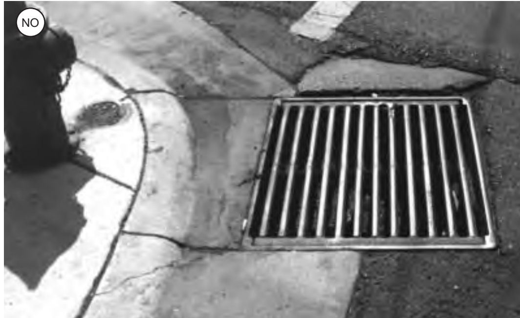
Figure 2-14: This drainage grate has two main problems. First, its parallel bars and slots can trap a bike wheel. Second, it's located in a likely path of a turning bicyclist.
