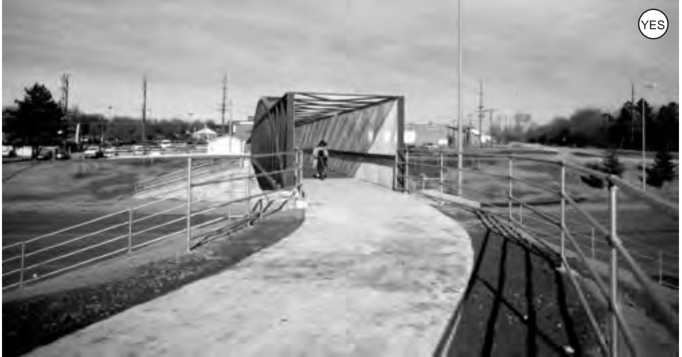
Figure 4-90: Existing grade differences made it relatively easy to carry this rail-trail above a major suburban arterial street.
