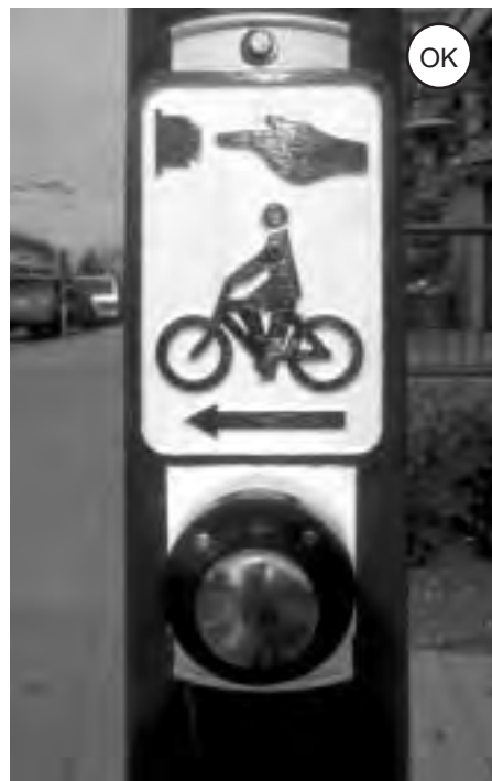
Figure 4-104: Path users need a way to trip the signal. If a loop detector is used for bicyclists, a push button for pedestrians should also be provided. Alternative means of detection (e.g., infrared) have been used for such purposes.
