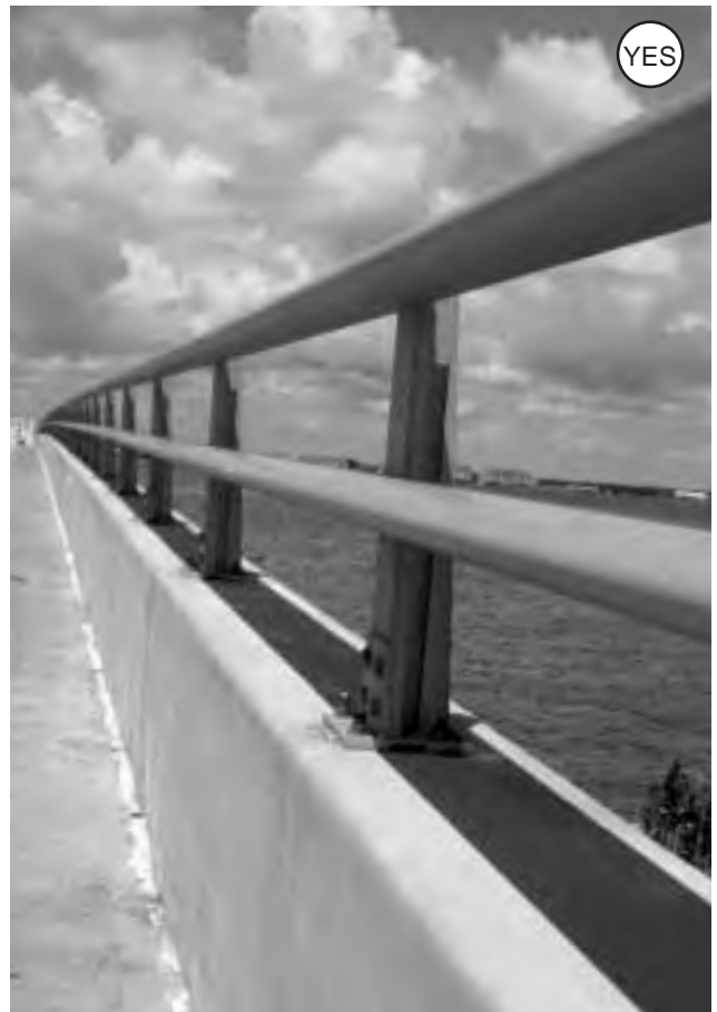
Figure 2-57: This bridge has a 54 in. railing that protects bicyclists from going over the top and into the river. Although a low-probability event, the consequences would be severe.
