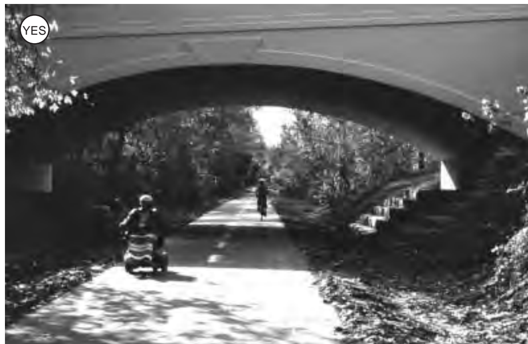
Figure 4-117: An open and airy underpass. Note the generous clearances on either side.
