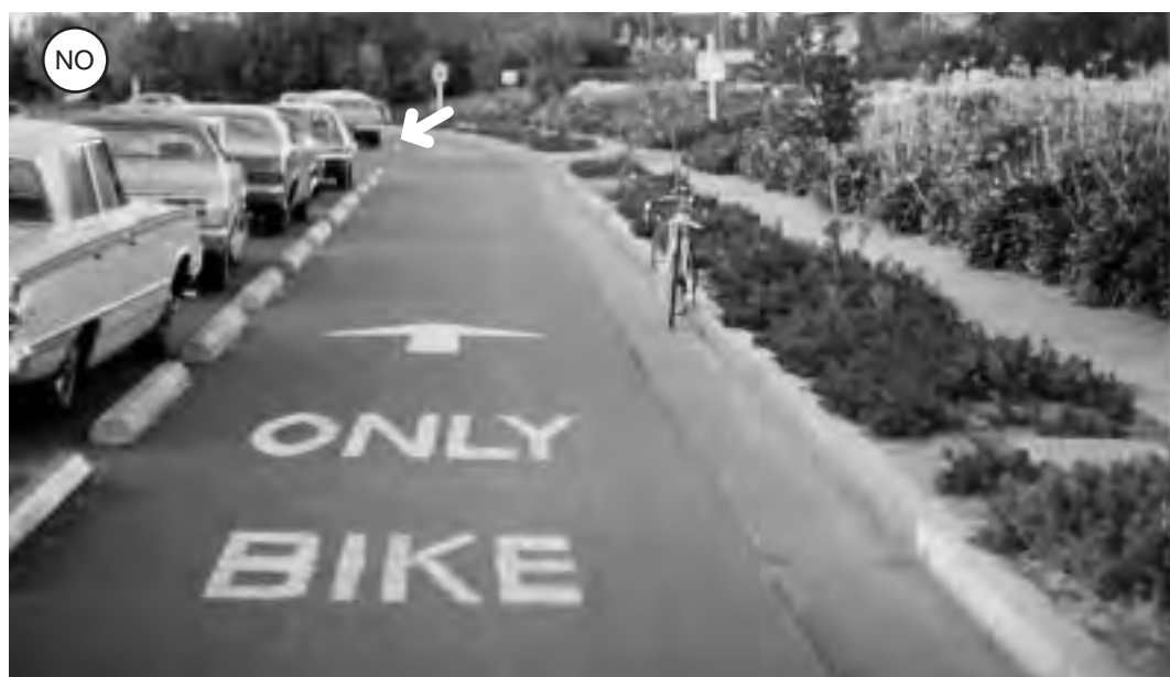
Fig. 3-5: A bicycle lane to the right of parked cars creates sight obstructions, keeping bicyclists and turning motorists from seeing each other. This is particularly dangerous at intersections and driveways (see arrow). In addition, crossing pedestrians may not notice – or be noticed by – bicyclists.
