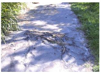
Photo 8.8 Example tree root damage to an off-road path. Near Malabar Rd, Malabar.
