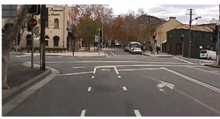
Photo 7.7: Example of bicycle lanes through a signalised intersection. Union St, Ultimo.
