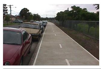
Photo 8.1 (Left top): Example of a reinforced concrete path with an asphalt wearing course. Running track adjacent is compressed granite with concrete edging. The Bay Run Cycleway, King Georges Park, Rozelle. Photo 8.2 (Left bottom): Example of a reinforced concrete shared path. This path has been continuously poured with transverse saw cut contraction joints at 3m intervals. Broomfield St, Cabramatta.
