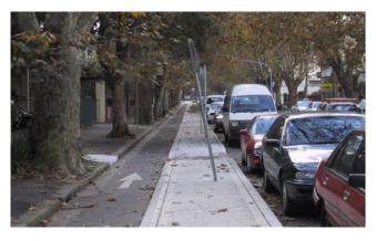
Photo 5.9 (above): Protected bicycle contraflow lane located to the kerbside of parallel car parking. Bourke St, Surry Hills.
