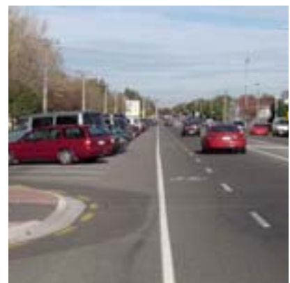
Cycle lane outside angle parking, Greers Road, Christchurch, New Zealand. Note: clearance is barely sufficient. (Photo: Tim Hughes)
