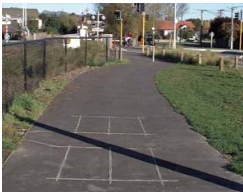
Detector loops on railway cycle path, Christchurch, New Zealand. (Photo: Axel Wilke)
