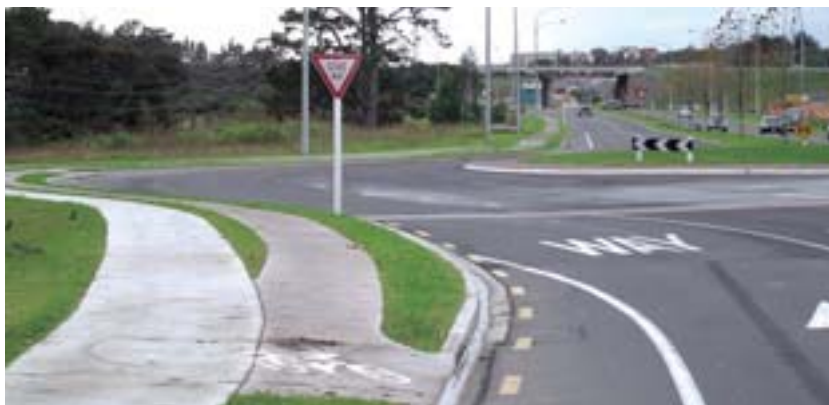
Cycle lane diverts to cycle path to negotiate multi-lane roundabout, Otaha Valley Road, Albany, New Zealand. (Photo: Tim Hughes)
