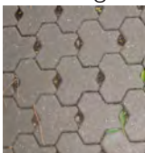
Permeable Paving
