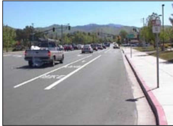
Figure 5.15 - This bike lane protects bicyclists from right turning automobiles at the intersection
