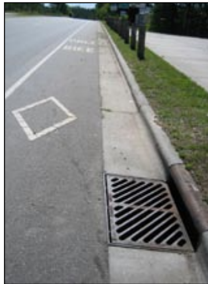
Figure 5.65 - New Bicycle Friendly Drainage Grate on Martin Luther King Blvd in Durham
