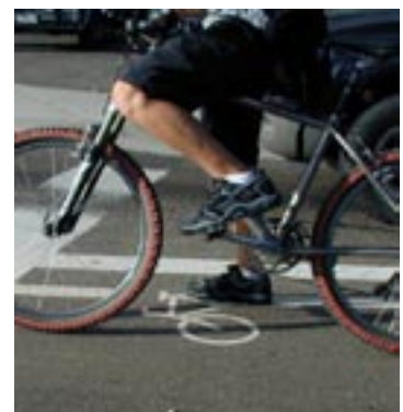
Figure 5.22 - Appropriate pavement marking to aid bicyclists in locating loop detectors at intersections
