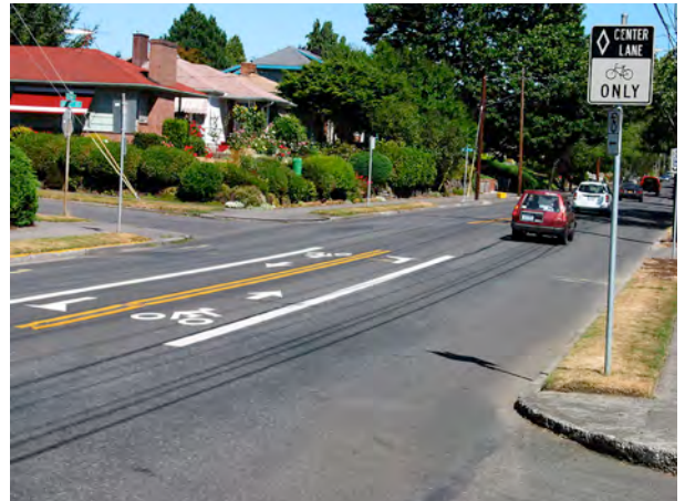
Two Way Center Left Turn - Portland, Oregon
