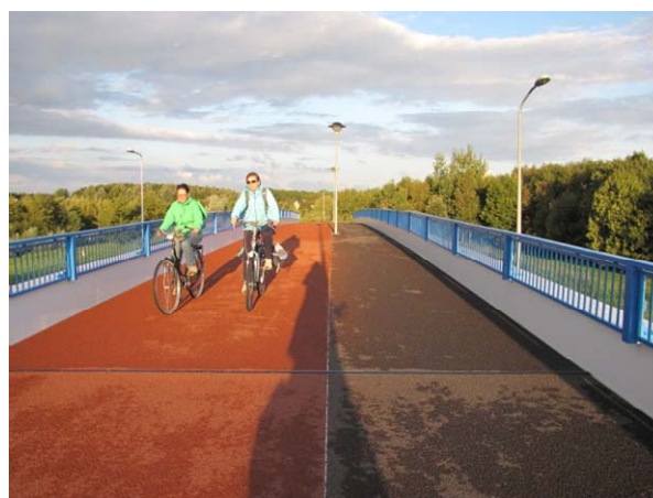
Figure 4-26: NMT Bridge (Lelystad)
