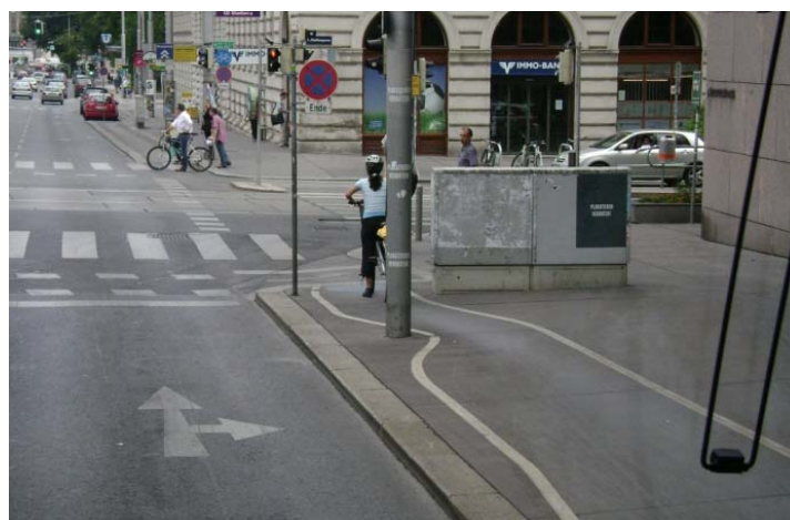
Figure 5-2: RM 1 Line Marking Highlighting Obstruction
