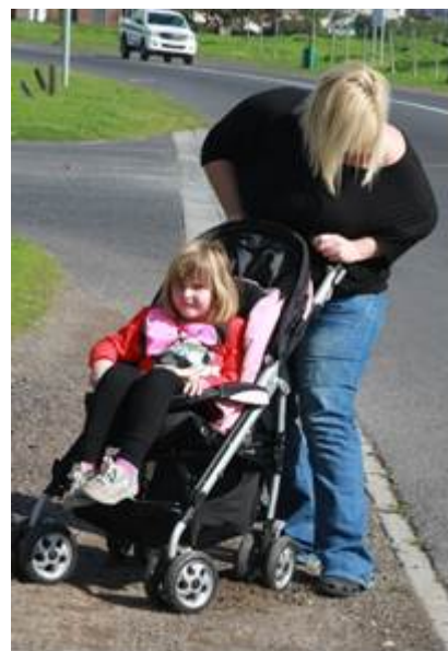
Figure 9-2: Push Cart Stuck in Small Surface Defect
