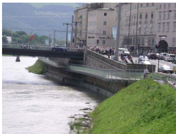
Figure 4-25: Bicycle Lane Under Bridge (Salzburg)
