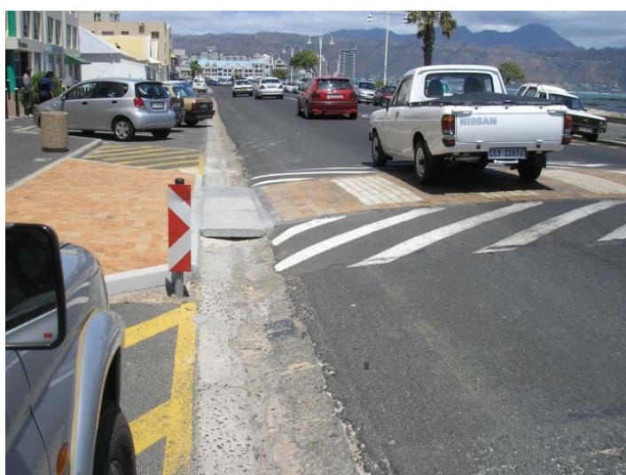
Figure 5-5: Drainage and Access for People in Wheelchairs Provided (Cape Town)
