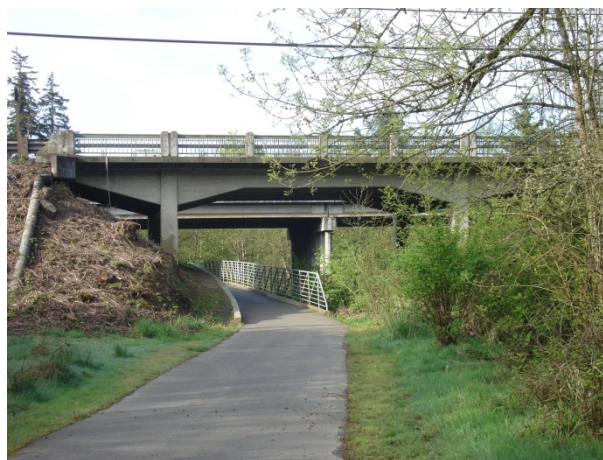
Figure 4-8: NMT Underpass Using River Bridge
