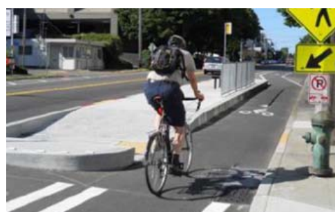
Figure 6-4: Bus Access Gap Reduction
