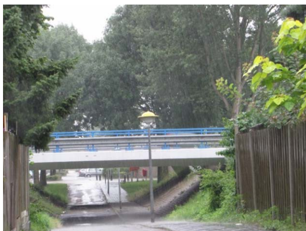
Figure 4-28: NMT Underpass (Lelystad)
