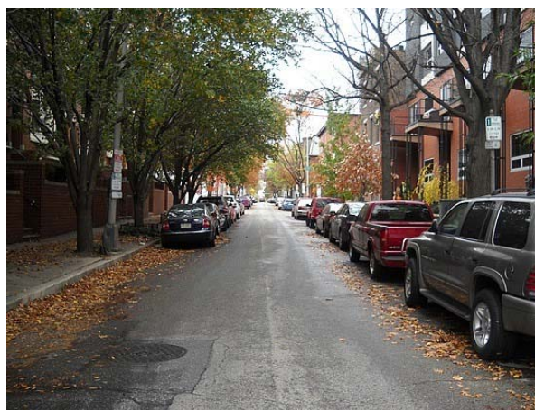
Figure 4-22: Access Road (Miami)
