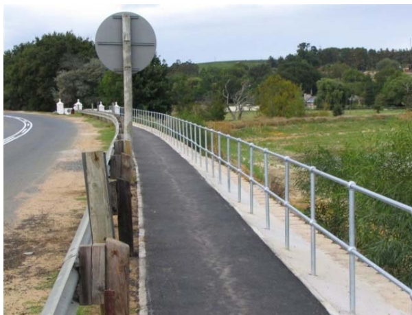
Figure 4-13: Walkway behind Guardrail with Light Barrier on High Fill
