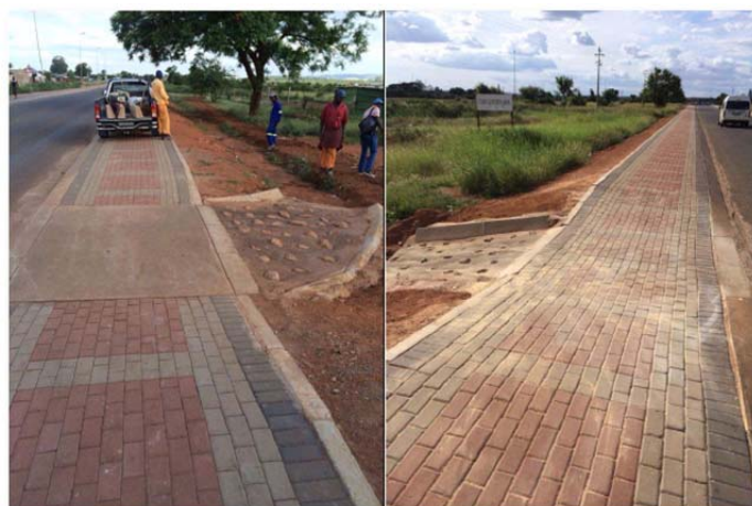
Figure 4-7: Good Drainage Along a Sidewalk
