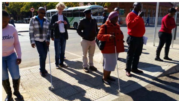
Figure 4-34: Tactile Paving at Dropped Midblock Facility
