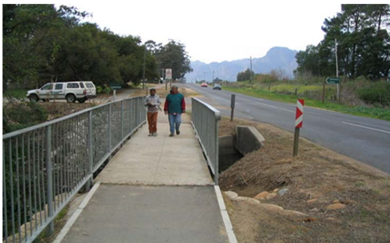
Example of a separate NMT bridge structure next to the roadway
