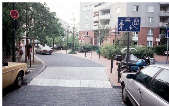
Figure 5-4: Example of a Good Speed Table (Germany)
