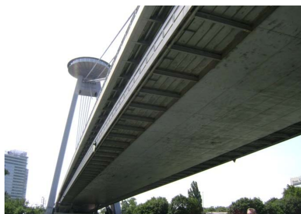
Figure 4-12: Walkway below Highway Bridge (Bratislava)
