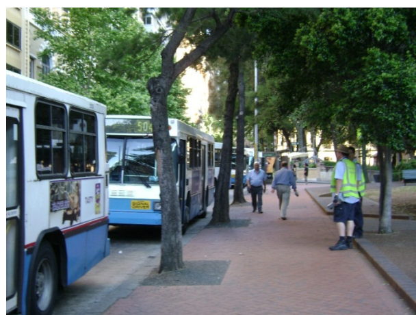
Figure 9-4: Tree Boles Protected with Asphalt (Sydney)
