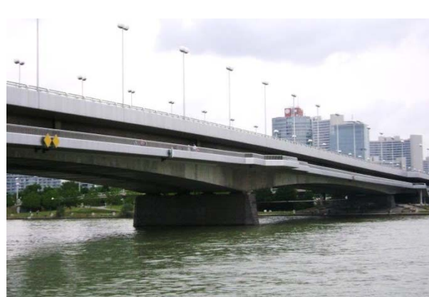
Figure 4-11: Walkway Suspended on Highway Bridge (Vienna)
