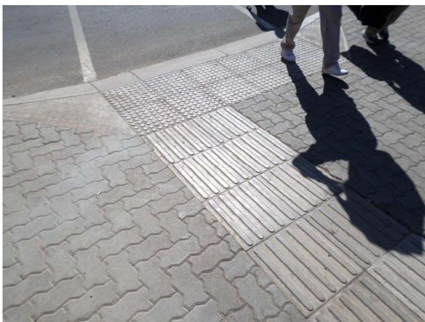
Figure 5-8: Guidance and Directional Tactile Pavers
