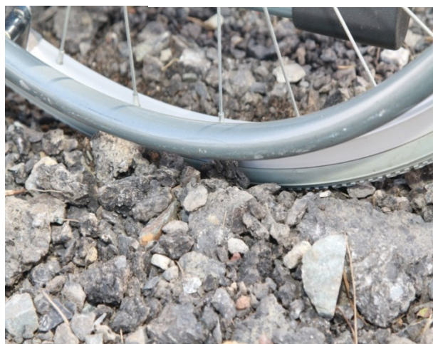
Figure 9-3: Wheelchair Punctured by Loose Stones
