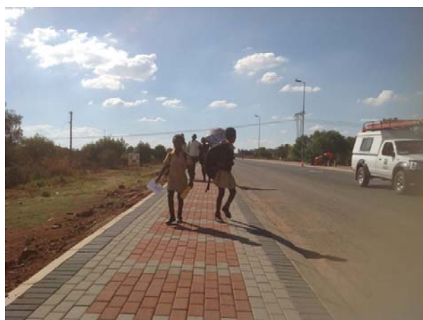
Figure 4-23: Access Road (Soshanguve, City of Tshwane)
