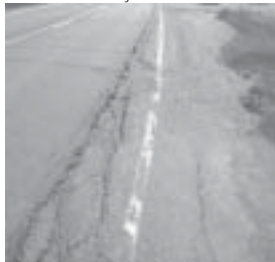
When resurfacing occurs over old concrete roadways, longitudinal cracks may appear where bicyclists normally ride.
