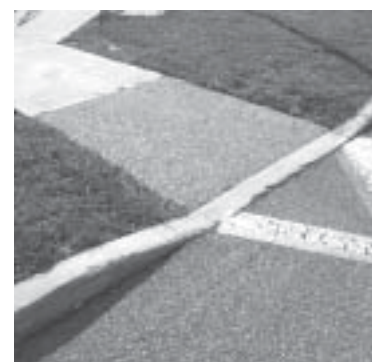
The use of grooved concrete or exposed aggregate should not be relied upon to warn pedestrians of potentially hazardous situations, such as ramps.
