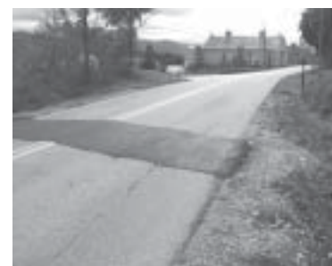
Backfill and compact utility cuts so that the cut will be flush with the existing surface.
