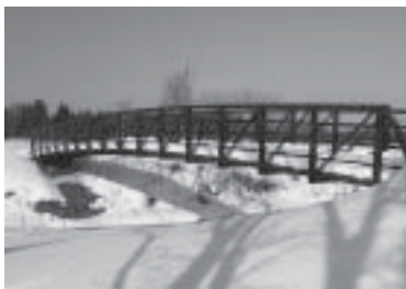
Many trails use prefabricated bridges, which are pre-engineered, constructed off-site, delivered to the site by the manufacturer, and lifted onto appropriate footings by a crane.
