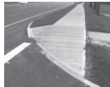
Ramps and landings that lead directly to the roadway should have a surface that is finished with a heavy broomed pattern perpendicular to the direction of travel in addition to truncated domes at the base of the ramp.
