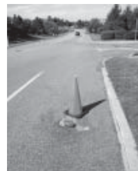
Remove uneven edges and grooves around utility covers and utility cuts.
