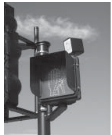
Auditory pedestrian signals may be provided when the need is established and an engineering analysis indicates the installation will add to the safety of pedestrians.
