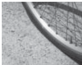
Aggregate suitable for all bikes and wheelchairs. Youghiogheny Trail, Ohio, Pennsylvania.
