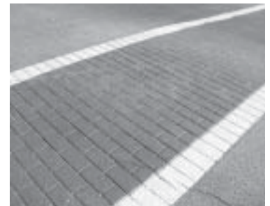
Textured crosswalks provide drivers with visual and audible clues that they are in a pedestrian environment.
