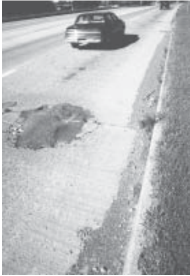
Small bumps and cracks that are barely noticeable to motor vehicles can cause a bicycle to crash or swerve.
