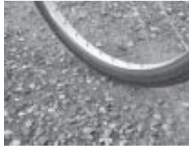
Aggregate too large for any use. Beebe Spur Rail Trail, Newport, Vermont (before replacement)
