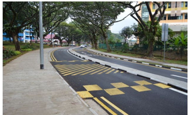
After: Bus-friendly Hump implemented along with centre divider at Jurong West Street 52
