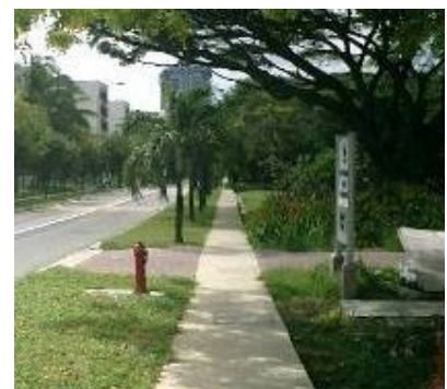
ABOVE: Roadside drain reconstructed as box drain which doubled up as footpath
