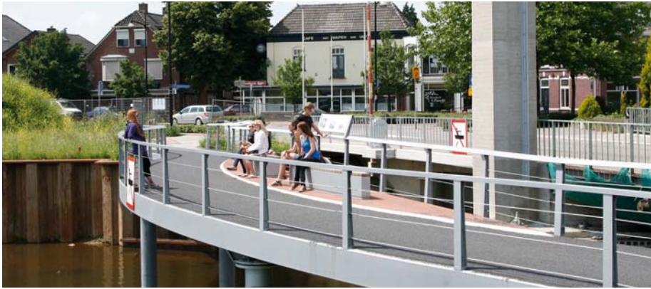
Figure 1.5 Ulfth bicycle and pedestrian bridge Curved layout offers room for benches, adding a function to the bridge
