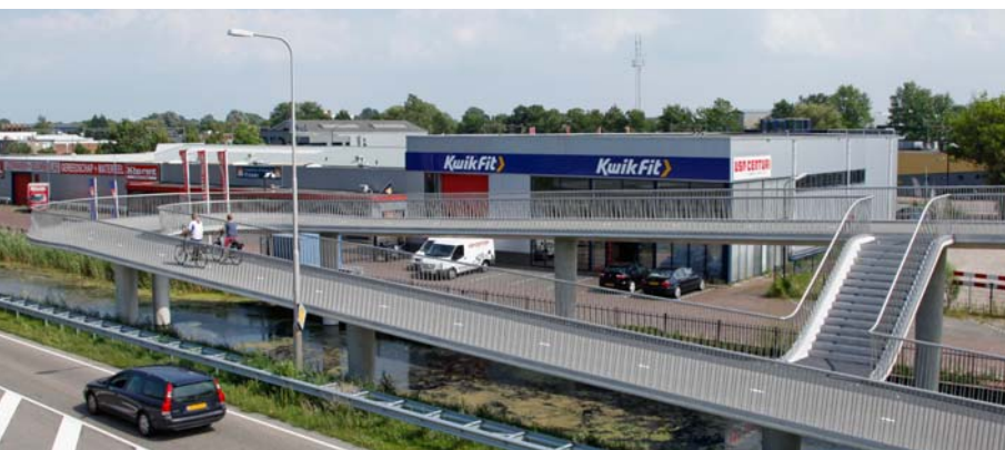
Figure 1.2 Bicycle bridge Heerhugowaard Businesses remain clearly visible due to slender bridge design and transparent railing
