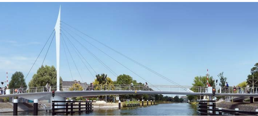
Figure 7.7 Swing bridge Rijswijk The bridge's horizontal clearance equals the width of the canal
