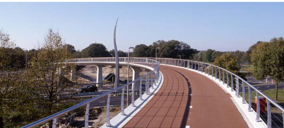
Figure 7.5 Auke Vleerstraat Bridge Due to its length, the bridge has a gentle slope
