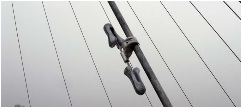
Figure 4.10 Tuned mass damper
