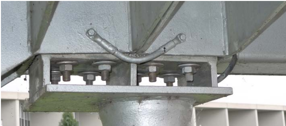
Figure 1.9 Nesseland Bridges Close-up of earthing system applied
