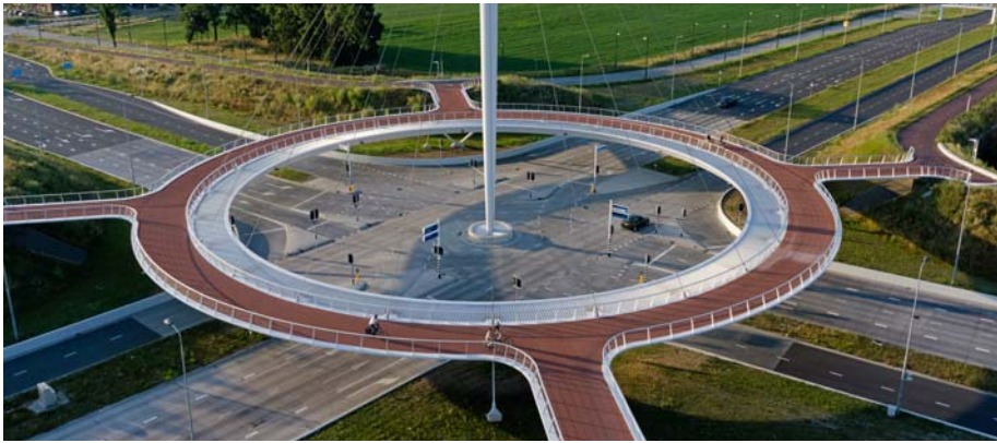
Figure 1.7 Hovenring Lowering the intersection underneath allowed for comfortable slopes
