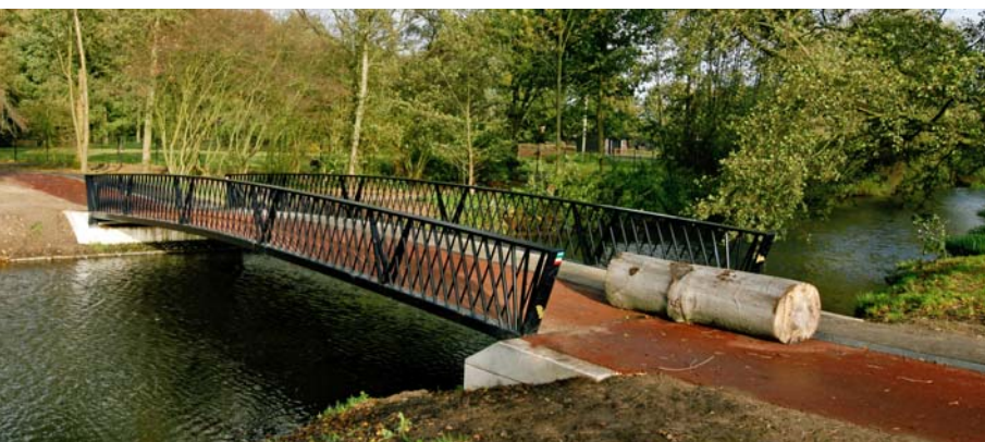
Figure 4.4 Vehicle obstruction Not so ordinary but effective solution to obstruct vehicle access
