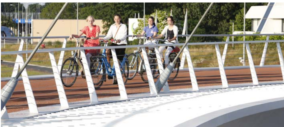
Figure 7.2 Hovenring Cable anchorage
