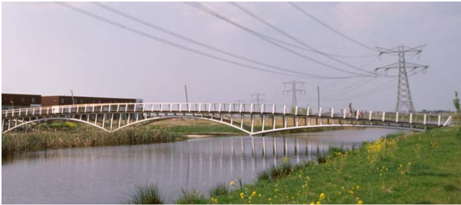
Figure 1.8 Nesseland Bridges Overhead power lines meant the steel bridges had to be earthed
