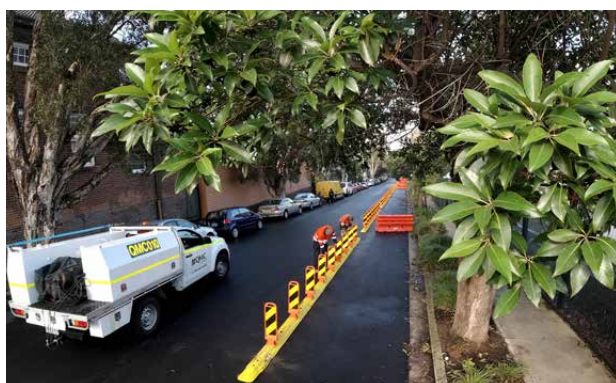
Figure 6.3 Installing the infrastructure required to support a pop-up cycleway is relatively quick and simple, as demonstrated on Henderson Road (Credit: Transport for NSW)
