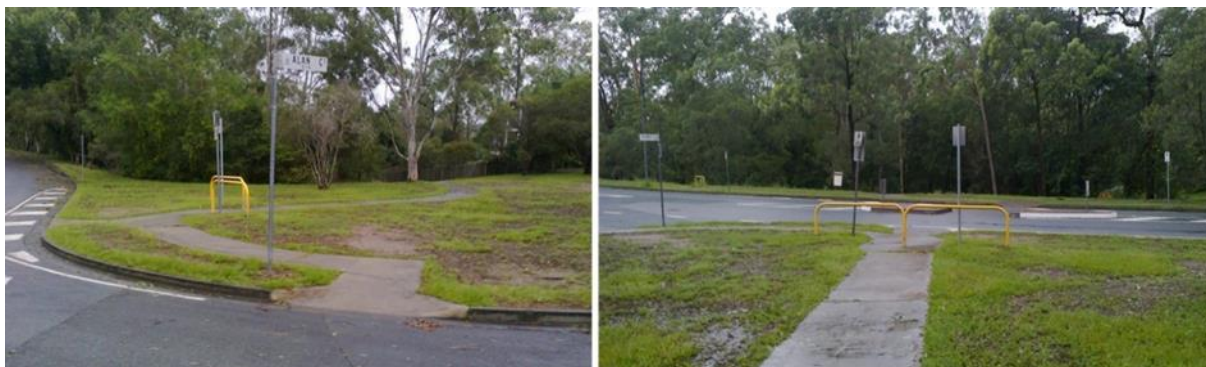
Figure C.4 – Redundant U-rail type terminal barrier
