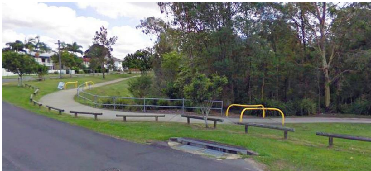
Figure C.2 – Excessive use of physical barriers to slow people riding bikes on approach to a blind corner
