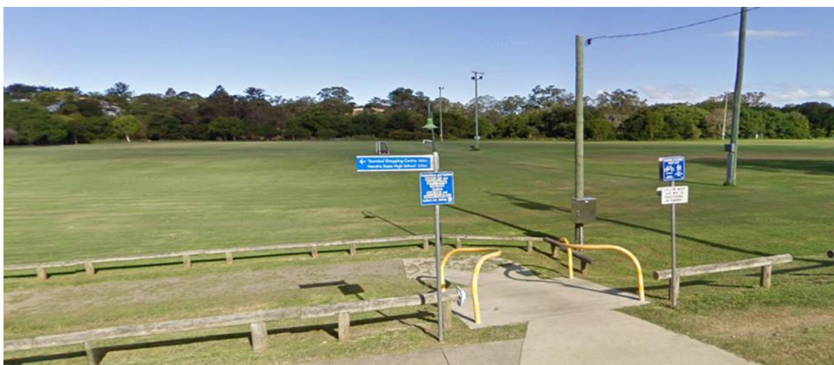
Figure C.6 – Hazardous positioning of a path terminal barrier
