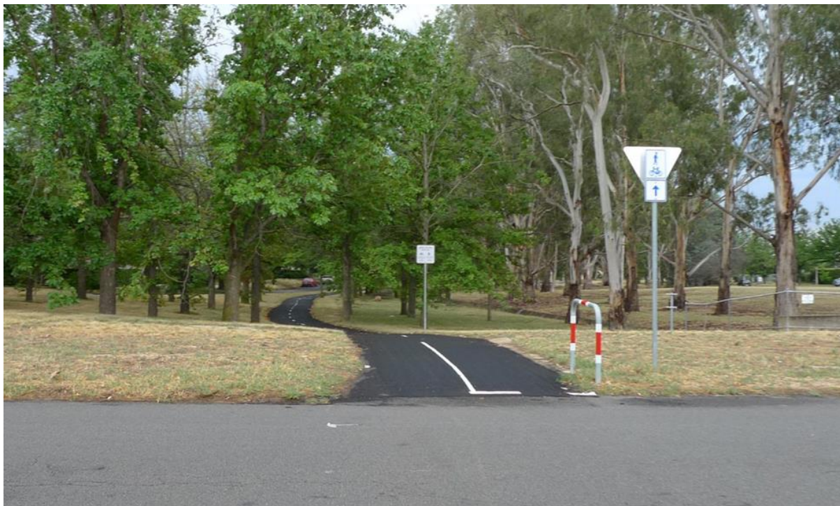
Figure C.1 – Path with minimal termination treatment
