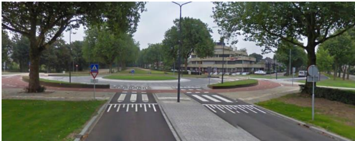
Figure 4.4(A) – Single-lane roundabout, motor vehicle entry and exit angle 90°, two-way cycle track with raised priority crossings and zebra crossings for pedestrian priority, Den Bosch, The Netherlands (LTS1)
