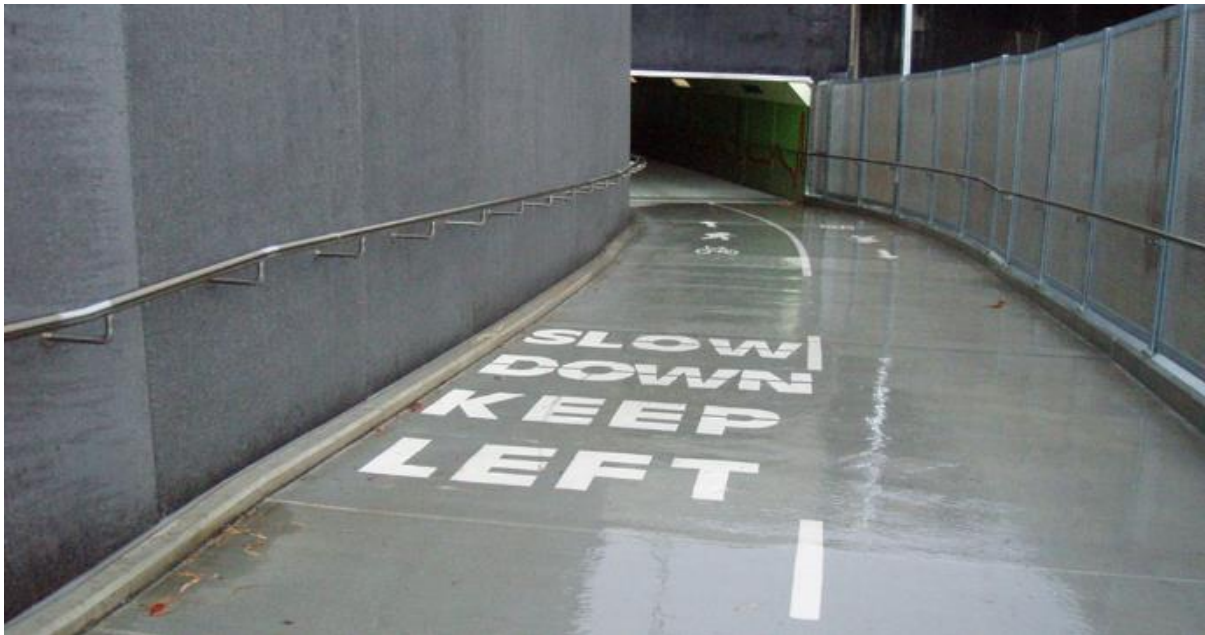
Figure 3.5(b) – Pavement markings use on a sight restricted corner to manage approach speed
