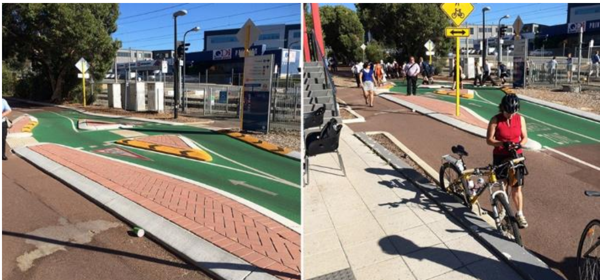
Figure 3.5(c) – Shared path slow point treatment at railway station access point
