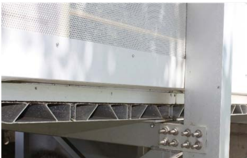
Figure 15.3(c) - Section through aluminium deck panels at Aeroglen
