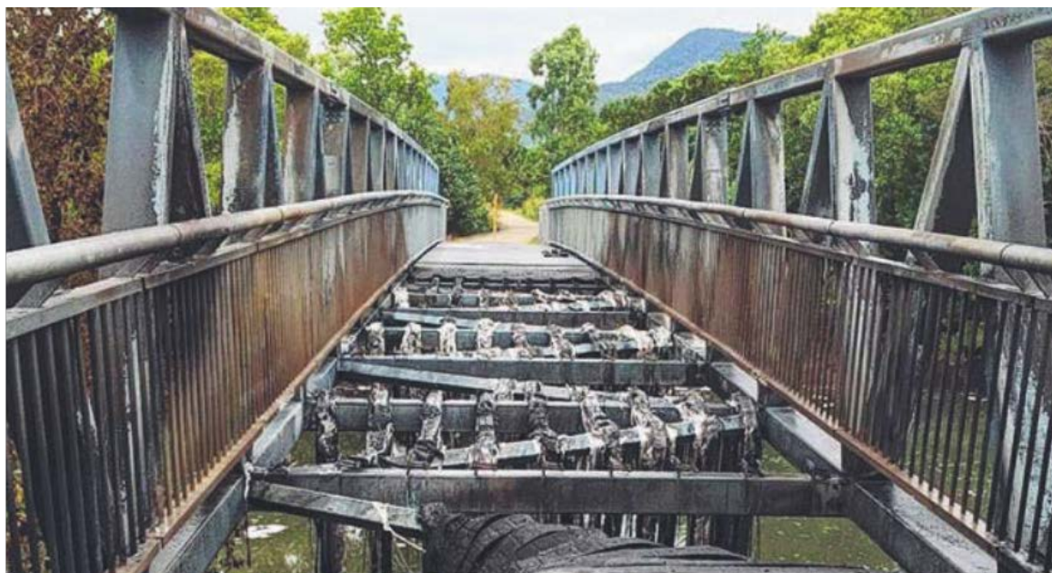
Figure 13.8(a) - Fire damage to recycled plastic deck
