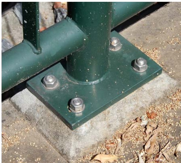
Figure 13.3(d) - Stainless steel hold down bolts
