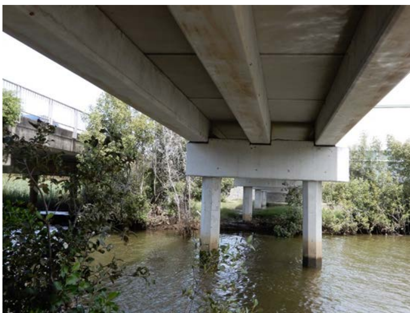
Figure 14.4.1 - Girder arrangement at Schulz Canal shared use bridge
