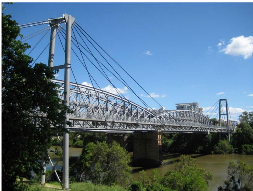
Figure 14.8 - Jack Pesch cable stayed bridge at Indooroopilly
