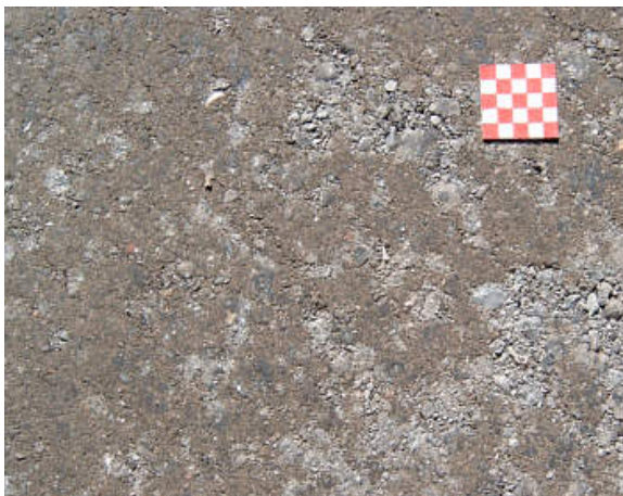
Foamed bitumen path with added cement.
