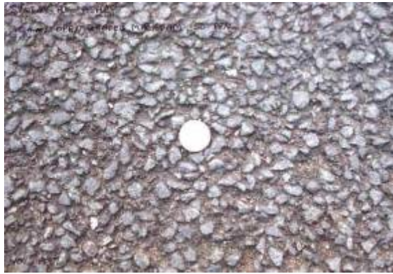
Clogged pores due to dust and mud
