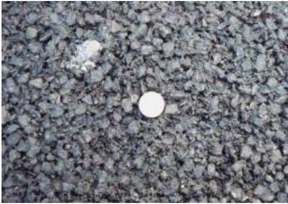
Open pores (fresh porous asphalt)
