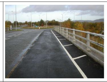
Bothwell Bridge over the A725 dual carriageway north of Hamilton. The parapet height is 1.1m and white lines have been used to pull the cyclists away from the parapet edge and so the safety auditors deemed no parapet works were necessary. The route is an unsegregated shared use section of path on NCN 74.
