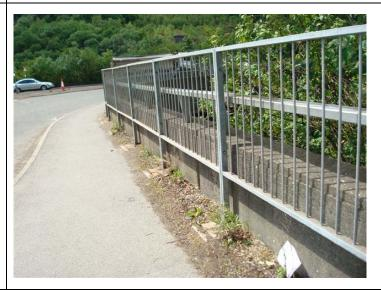
Havering: raised pedestrian guard railing undertaken because the council felt that there was a significant drop from the edge of the path into an adjacent watercourse.
