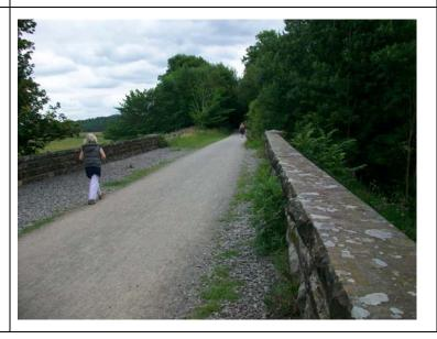
Bristol: whilst not a bridge, the 'Chocolate Path' alongside River Avon has a 970mm parapet height.
