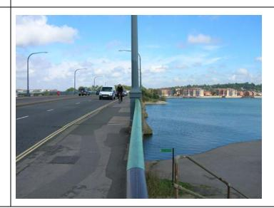
Bristol: signed cycle route on bridge over M32. Parapet height 1.1m
