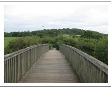
Port Talbot: Connect2 route using old aqueduct with 1.3m high parapets
