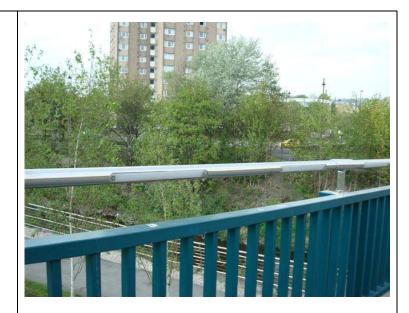
Taff Trail over a trunk road near Taffs Well: pedestrian guardrailing installed in front of existing parapet.
