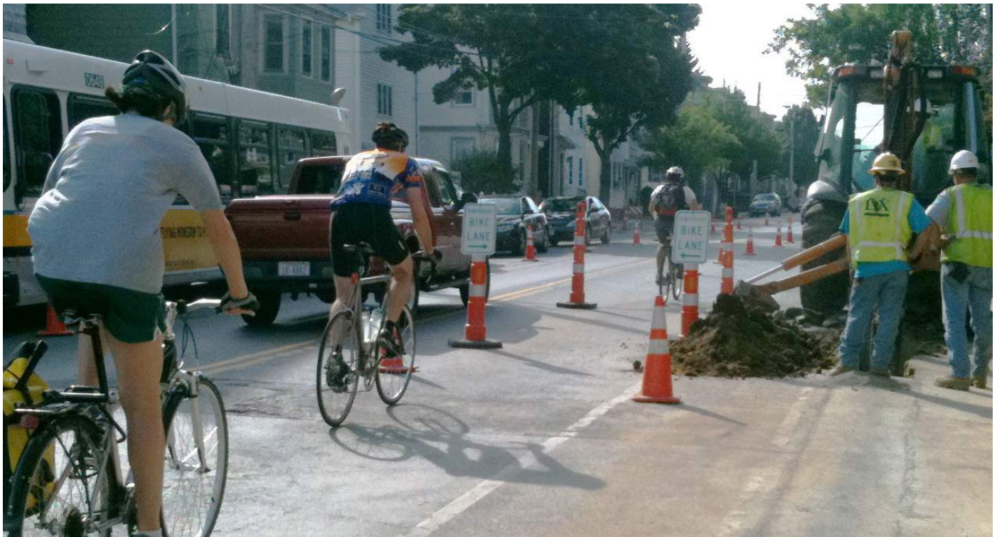
Figure 9.5: Construction zone featuring temporary bike lane.
