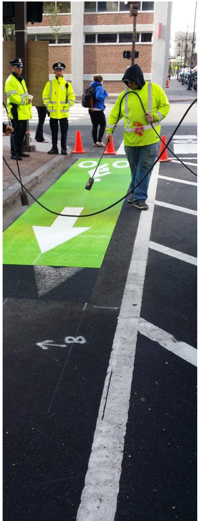
Figure 9.6: Construction crew installing bicycle decal and green pavement markings.
