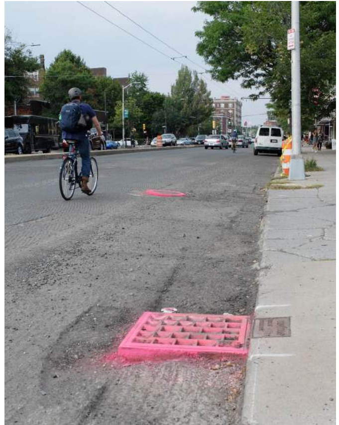
Figure 9.4: Street repaving zone featuring manholes painted with reflective pink paint.
