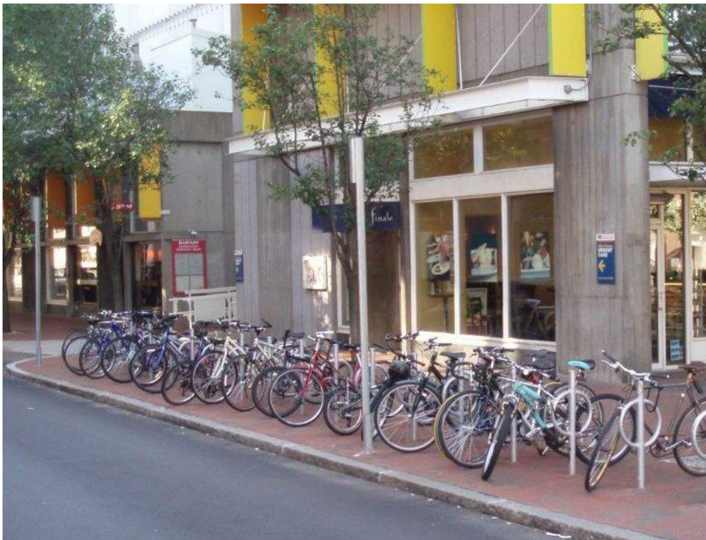
Figure 7.3: Curb extensions are sometimes built in order to provide space for added bicycle parking, and the “post and ring” model has a compact footprint.
