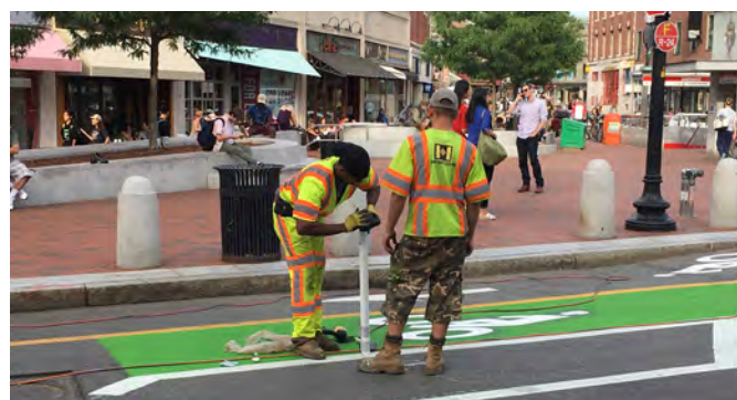
Installation of a new flex post on a separated bike lane.
