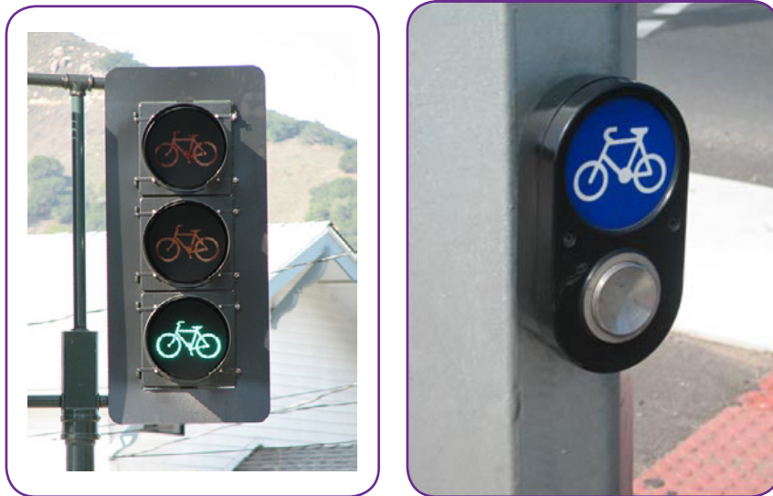
Figure 3-12 Dedicated Bicycle Signals and Signal Phases
