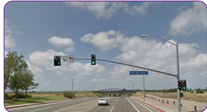
Figure 4-4 Placentia Avenue at Fairview Park with buffered bicycle lanes and multi-use trail bridge
