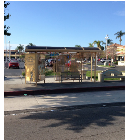
Figure 4-18 Sheltered Bus Stop
