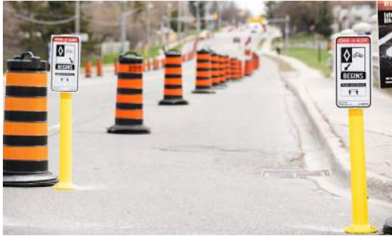
Figure 19 | Temporary vertical separation created by plastic traffic barrels protects cyclists from injury if they hit the barrier (Brampton, Ontario)
