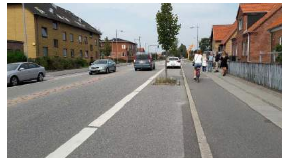
Figure 10 | In Nykøbing F, Denmark, a bicycle lane is located next to the sidewalk and separated from the vehicle lane by a parking lane and a curbstone
