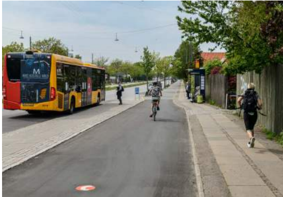
Figure 36 | Permanent cycle track with bus stop and parking on a bicycle superhighway in Copenhagen
