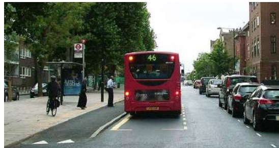
Figure 33 | Copenhagen-style bus stop in London, where bike lane is elevated and markings indicate that cyclists must yield to passengers
