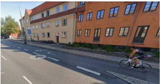
Figure 28 | A bike lane buffer zone ending, allowing for bikes and turning traffic to mix prior to the intersection, Denmark
