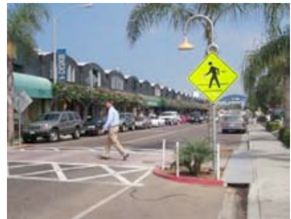
4S) Raised crosswalks (speed tables) provide clear signs of a pedestrian crossing but need to be limited to lower speed, lower volume streets. Photo credit: Andy Hamilton
