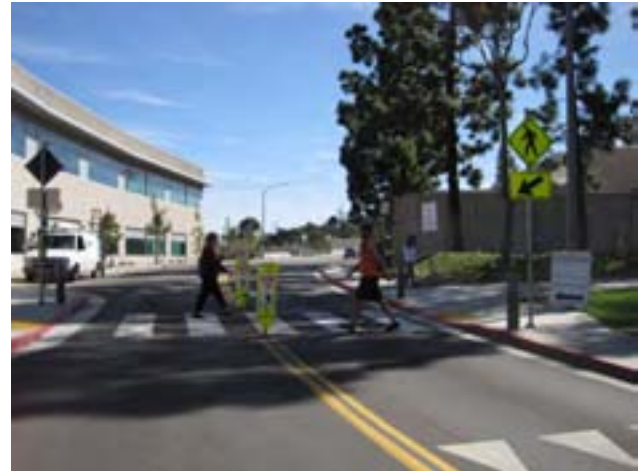
13S) The response time for stopping traffic for this mid-block crossing was quick. The design of the adjacent walkways concentrated pedestrians into this walkway crossing. Photo credit: Joe Punsalan
