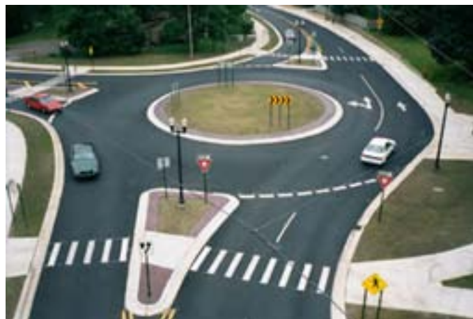
18S) Modern roundabout with properly planned pedestrian crossings, markings, signage and lighting. Photo credit: Dan Burden
