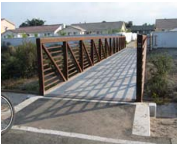
6C) Grade separated pedestrian crossings should generally be avoided because of the expense and low level of use. Some circumstances warrant their use such as over freeways, railroads and other intensive surface uses where at-grade crossing may not be safe. Bridges that limit the amount of vertical climbing or do not go dramatically out of direction, will be used. Photo credit: Joe Punsalan
