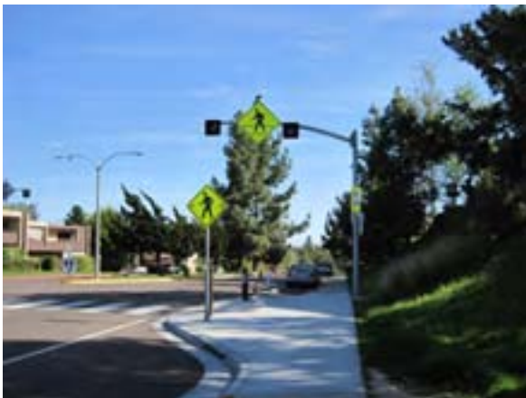
5S) Adequate lighting, pop-outs, the latest MUTCD approved signs and high visibility markings are essential for non-controlled multi-lane mid-block crossings. Note the stop bar should be located at least 15 feet from the actual crosswalk (see image on right). Photo credit above: Joe Punsalan
