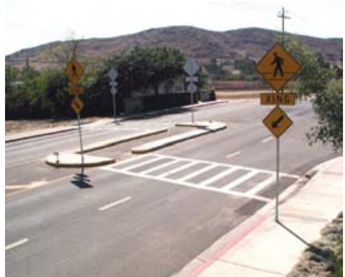
1S) Median refuges are essential where mid-block crossings are contemplated. They can include a straight cut-through or a staggered or coral style crossing. Photo credit: Dan Burden
