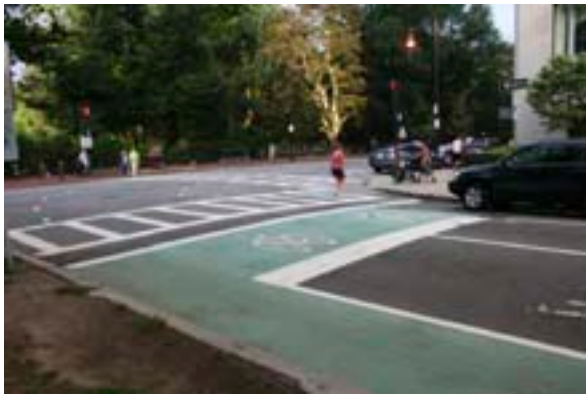
7B) A bike box creates an advanced stop bar for cyclists. This extra room provides an area for cyclists to cue up in front of cars waiting at red light. While this treatment is still considered experimental by the MUTCD, it is thought that the treatment increases a bicyclist's visibility and therefore safety. Photo credit: Michael Singleton
