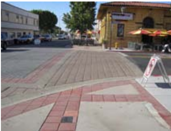
3S) Increased visibility can be obtained through a change of paving materials and striping. Photo credit: Joe Punsalan
