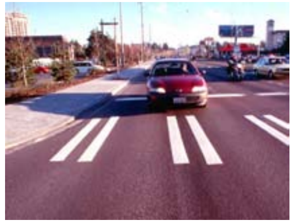
3S) Ladder style markings can be modified and spaced to lower the wear from vehicle tires. Photo credit: Dan Burden
