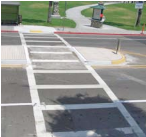
1S) A good example of a median refuge that provides access without ramps and protects a walker unable to make it across. Photo credit: Andy Hamilton
