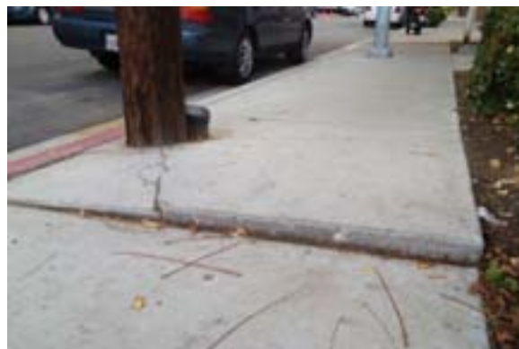
7A) Repair, slice or patch lifts on walk surfaces and/or reset ground level utility boxes to be flush. Photo credit: Joe Punsalan
