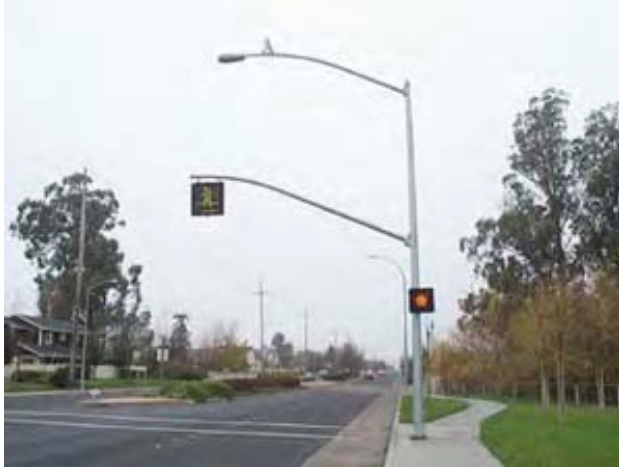
11S) This signal uses both a pedestrian crossing symbol as well as a red light when actuated. Photo credit: Michael Ronkin
