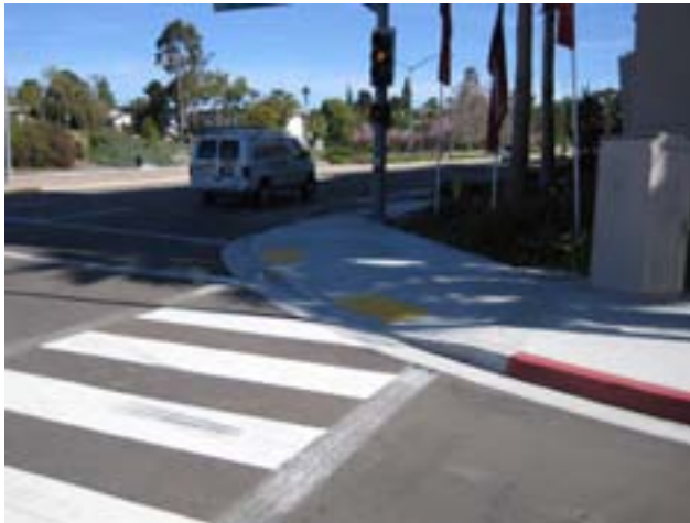
Perpendicular curb ramps at Trolley Ct. Photo Credit: Joe Punsalan
