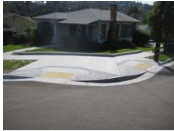
2S) Pedestrian pop-outs (curb extensions) can provide increased safety, improved visibility of pedestrians, protection for parked cars, and a shorter crossing distance for the pedestrian. They also provide for street furnishings, landscaping and social areas. Photo credit: Joe Punsalan
