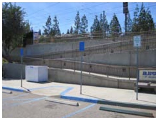
6C) To meet accessibility requirements, long ramps are required to access activity centers such as transit stations. Photo credit: Joe Punsalan
