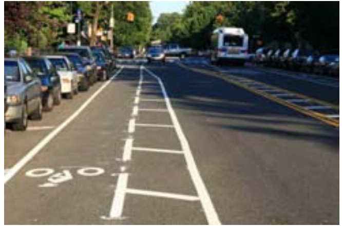
6B) A buffer removes extra space from a travel lane and increases the distance between vehicular and motor traffic. If the extra space is added to the bike lane and not diagonally striped, the bike lane can appear wide enough to be confused with a travel lane. Photo credit: APBP
