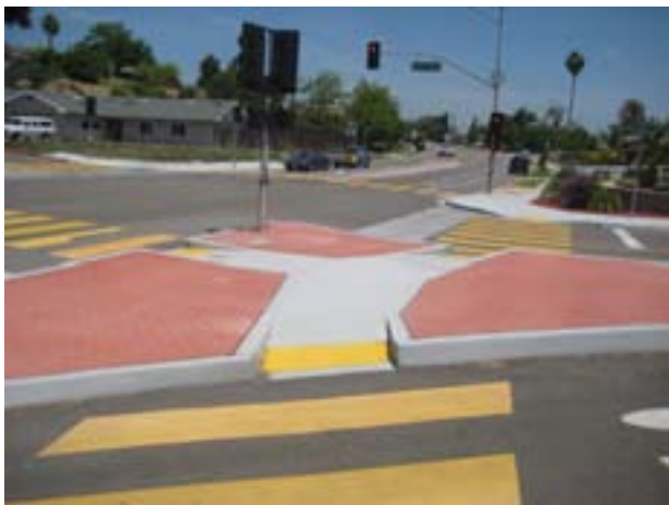
4C) Retrofitting wide streets and intersections to improve walkability, can be very expensive. It is generally far less expensive to build these streets with pedestrians and cyclists in mind than to retrofit later. Photo credit: Joe Punsalan
