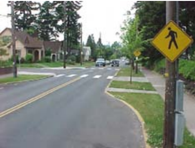
14S) This crossing is on a one lane in each direction street with curb extensions, striping, signage and trees that all help to slow a driver down. There is no multi-lane, multi-direction threat to this use of an uncontrolled mid-block crossing. Photo credit: Portland Office of Transportation
