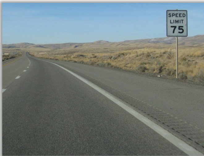
I-80: Although there is a rumble strip located adjacent to the fog line, wide shoulders provide adequate space for bicycles along this route.
