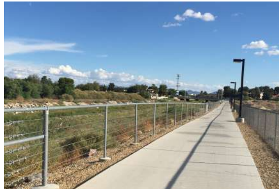
Figure 7.24: Bridge Structure Deck in Concrete to Reduce Maintenance
