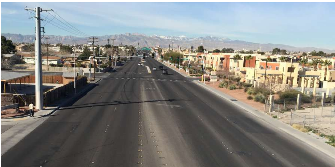
Figure 2.12: Cheyenne Ave features 12' travel lanes with 14' outside travel lanes
