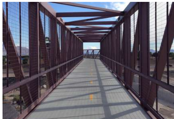
Figure 7.24: Bridge Structure Deck in Concrete to Reduce Maintenance
