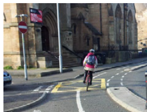
Yellow box marking reinforces cycle track priority at side road junction, Glasgow
