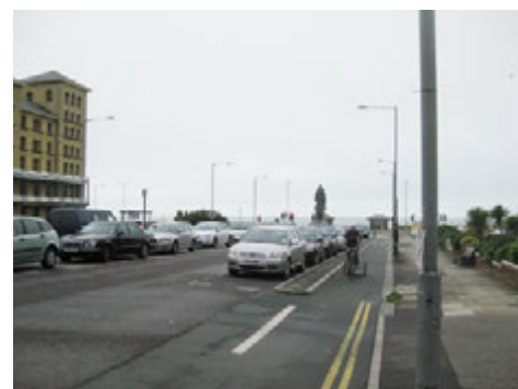
With-flow cycle track on the carriageway with wide kerb segregation adjacent to car parking, Brighton
