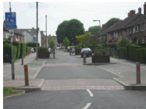
Home zone with relatively low cost treatment including flat-topped humps with sinusoidal ramps, Wilberforce Avenue, York
