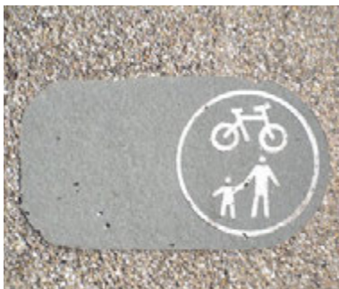
Low-key signage: adaptation of unsegregated shared use diagram 956 on track surface, Blackpool
