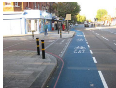
Advisory cycle lane across side road junction with entry treatment, Cycling Superhighway 7, London
