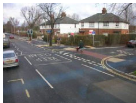
Existing residential estate road with reduced sight lines and insufficient space to bend out the cycle track by 5m. A 'partial priority' solution has been introduced whereby traffic exiting the side road gives way at the crossing, but vehicles entering retain priority. Oxford
