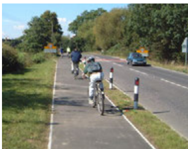
Rural unsegregated shared use track with verge forming margin strip. Note both the cycle track and margin strip are narrower than recommended for speed limits of 40mph or above
