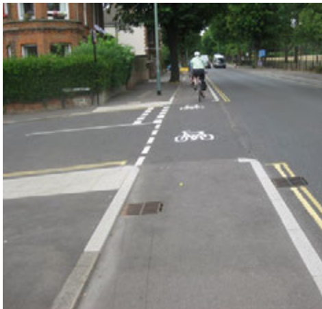
Cycle track with tight corner radii and no advisory lane markings at side road, Brighton
