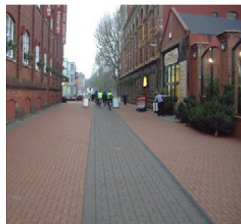
Use of contrasting materials to highlight cycling route through pedestrianised area, Bristol
