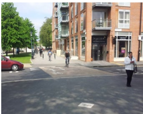
Unsegregated shared use route, with priority at crossing of side road. The crossing is set back 5m from a mini-roundabout (to left of photo) on a raised table, and retains the desire line for pedestrians and cyclists. The waiting vehicle has just exited the mini roundabout
