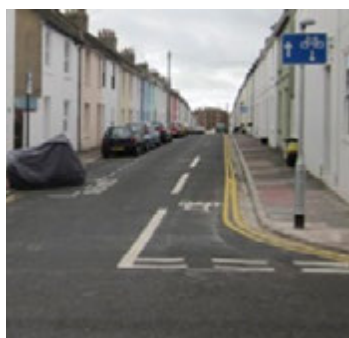
Vehicle entry (cycle exit) to one way street with contraflow cycling, Brighton
