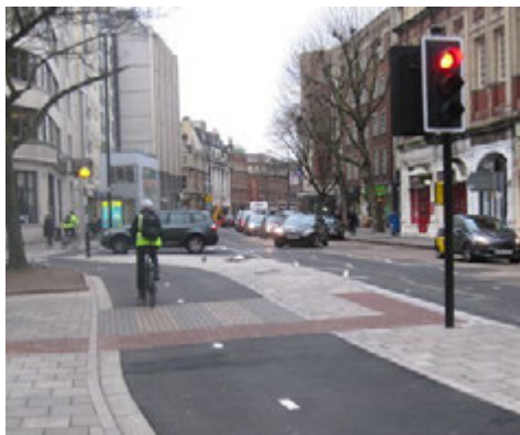
Segregated two-way track, formed by reallocating city centre traffic lane, Bristol - Note informal zebra crossing at Pelican crossing
