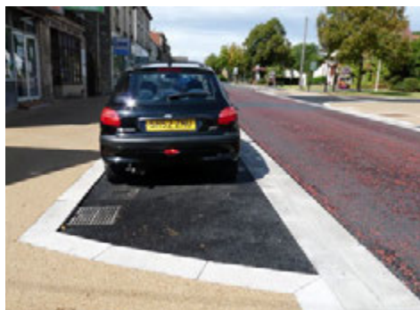
High street calmed with shared space principles: removal of centre line, reduction of carriageway width and reduction of kerb heights, Stonehouse, Gloucestershire
