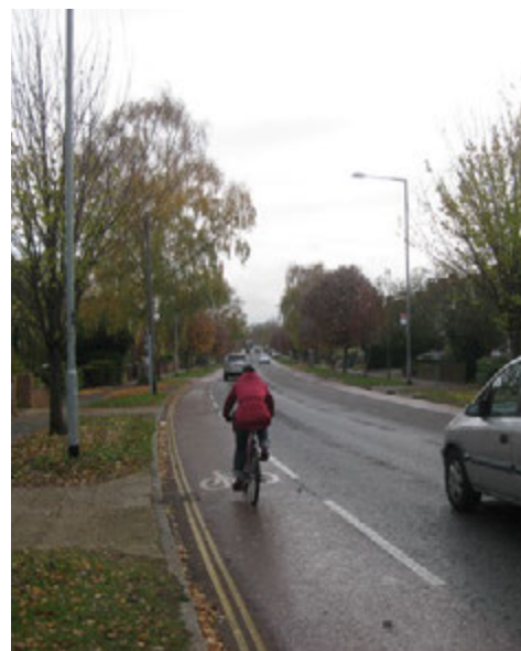
Centre line removed to allow advisory cycle lanes to be introduced, Cambridge
