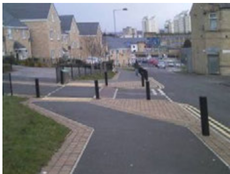
Unsegregated shared use track with raised informal crossing points in a new residential development. The tight junction radii and raised table ensure low vehicle speeds, which along with the low traffic volume, removes the need to mark priority for any one movement. Bradford
