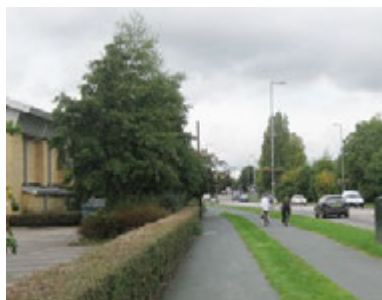
Segregated shared use with the form of segregation and the margin strip comprising a grass verge, Loughborough
