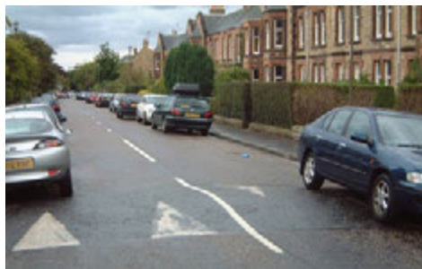
Sinusoidal road humps, Edinburgh
