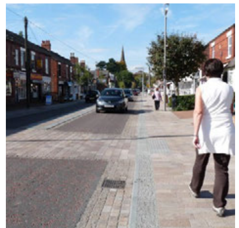
High street calmed with shared space principles: 2.0m traffic lanes with textured margin strips, a central median, reduced kerb heights and informal pedestrian crossings, Park Lane, Poynton
