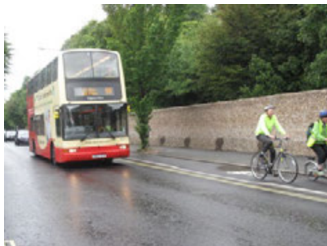
Hybrid cycle track showing mid link flush kerb to facilitate access to /from the carriageway. Old Shoreham Road, Brighton
