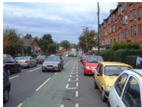
Hatched margin strip between with-flow advisory cycle lane and nearside parking bay, Glasgow
