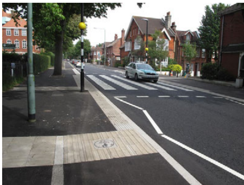
Hybrid tracks running into unsegregated pedestrian and cycle space at a 10m wide zebra crossing, Brighton
