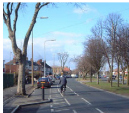
Removal of traffic lanes to provide cycle lanes, Hull
