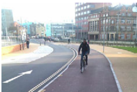
Segregated two-way hybrid track, formed by reallocating a city centre traffic lane, Leicester
