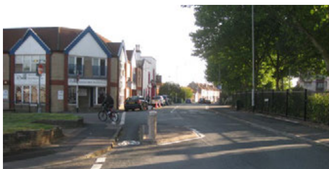
Cycle bypass at chicane, Bristol (left) and Shrewsbury (right). Note the bypass width is less than the recommended 1.5m minimum in both cases and would not accommodate a cycle trailer)
