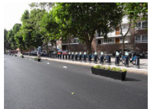
Light segregated cycle lane using Armadillos and planters, Camden London
