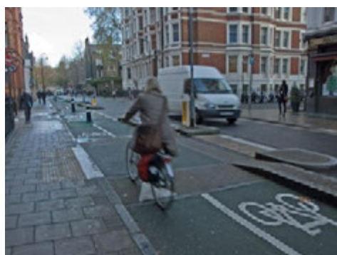
Cycle track raised to footway level and pedestrian refuge created to enable pedestrians to cross cycle track and traffic lanes separately, London
