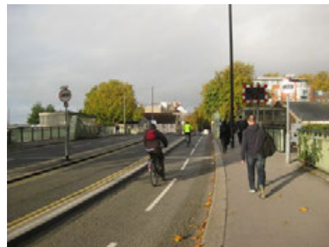
Two-way contraflow cycle track on the carriageway with kerb segregation, created by reallocation of one of two lanes on eastbound carriageway, Bristol
