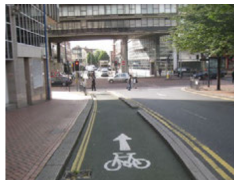
One-way contraflow cycle track on the carriageway with kerb segregation, Hill Street, Birmingham
