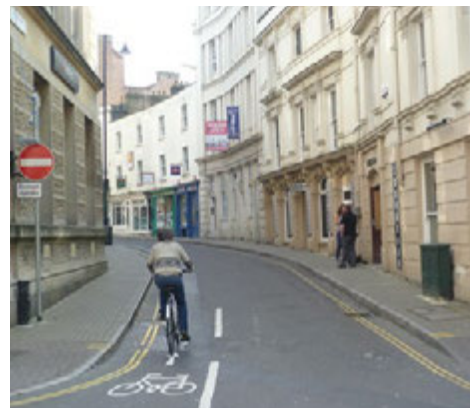
Vehicle exit (cycle entry) from one way street with unsegregated contraflow cycling, Bristol
