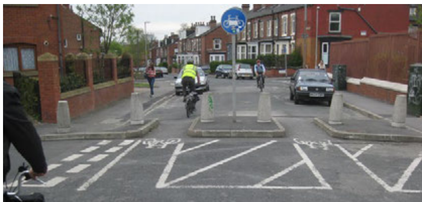
Two-way cycle exemption at a road closure, Leeds. This layout is more likely to be obstructed by parking on the far side of the closure, and the cycle gaps are less than the 1.5m recommended minimum
