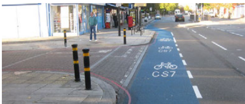
Advisory cycle lane across side road junction with entry treatment, Cycling Superhighway 7, London
