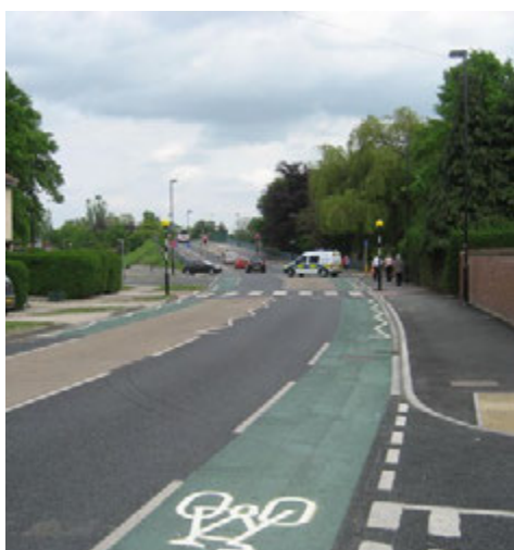
Coloured surfacing provides route continuity through pedestrian crossing zigzags, York
