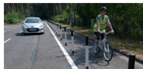
Light segregated cycle lane using wands
