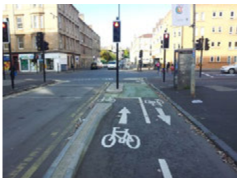
Two way cycle tracks increase complexity at signalised junctions and may require separate staging for cycle movements, Glasgow
