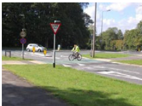
Shared use cycle track crossing set back from the junction on a raised table with priority over the minor arm; one of a package of priority crossings at side road junctions on key corridors in Scunthorpe
