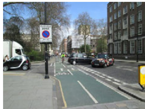
Use of coloured surfacing, diagram 1057 cycle symbols and diagram 1059 direction arrows at side road junction, London. The vehicle nudging out from a side road conceals an approaching cyclist from the taxi turning into the junction
