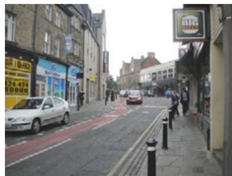
Contraflow cycling with advisory cycle lane and margin strip adjacent to parking bays, Penny Street, Lancaster. The contraflow cycle lane moves from the offside to the nearside of parking bays as it joins the heavily trafficked A6
