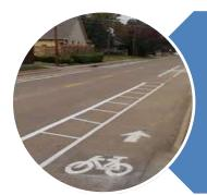
Buffered Bicycle Lanes (Class II) are implemented by painting or otherwise creating a flush buffer zone between a bicycle lane and the adjacent travel lane. While buffers are typically used between bicycle lanes and motor vehicle travel lanes, they may also be installed between bicycle lanes and parking lanes.
