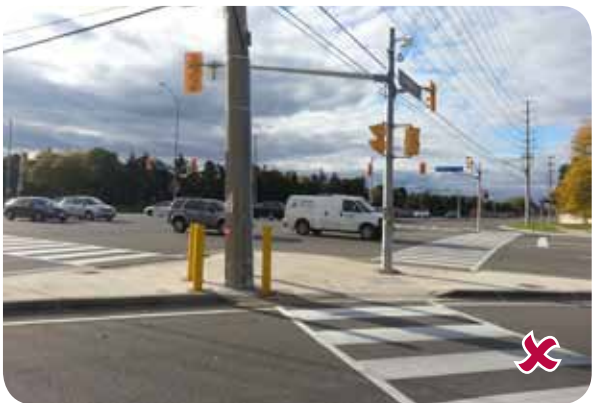
Removal of channelized right turn lanes
