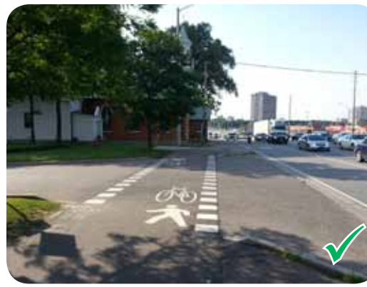
Pavement markings and geometry at driveways to slow traffic and improve visibility of cycling facilities, particularly multi-use trails
