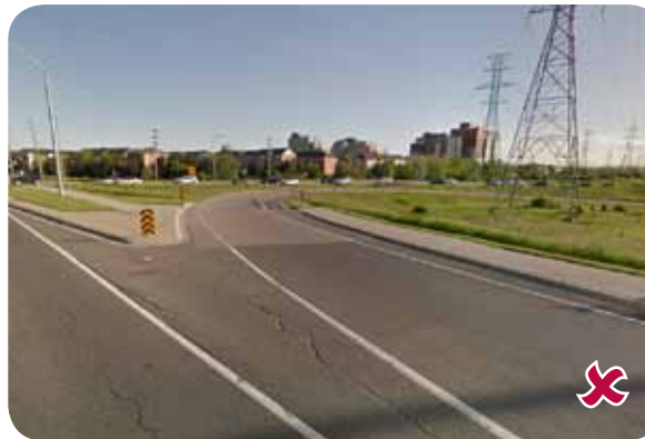
Reduced radii on highway ramps to slow down turning traffic at highway interchanges
