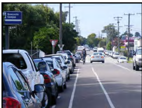
Chinchin St trial - narrowing of traffic lanes to provide bicycle lanes with separation to parked vehicles. Note that this treatment is no longer possible due to RMS requirements for minimum 1m safety strip.
