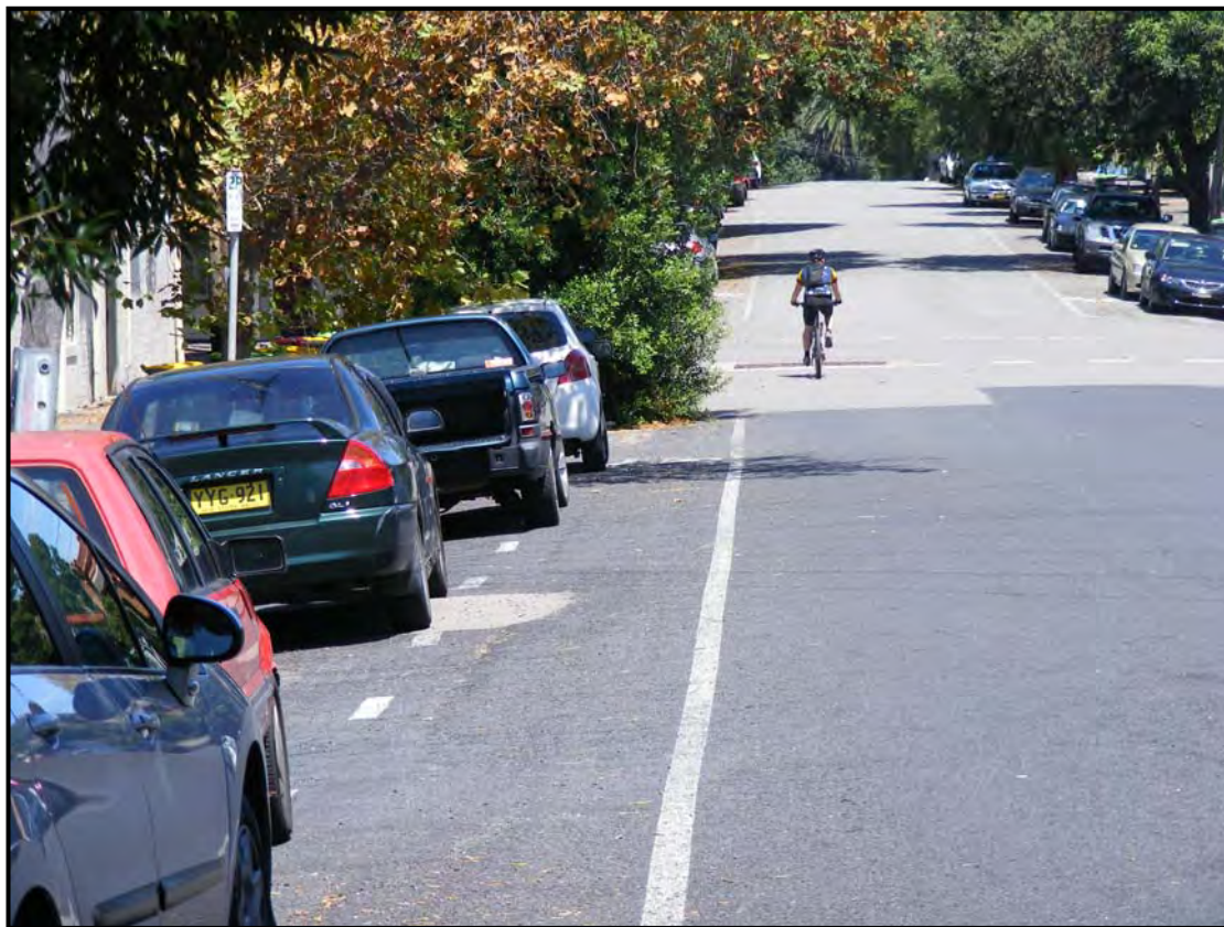
Example of bicycle shoulder lane, with rider demonstrating safer, more visible positioning away from the car door zone.
